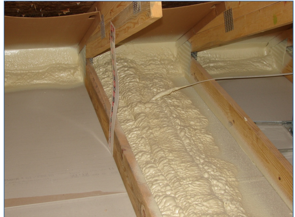
Sealed top plates of partition wall and exterior wall
