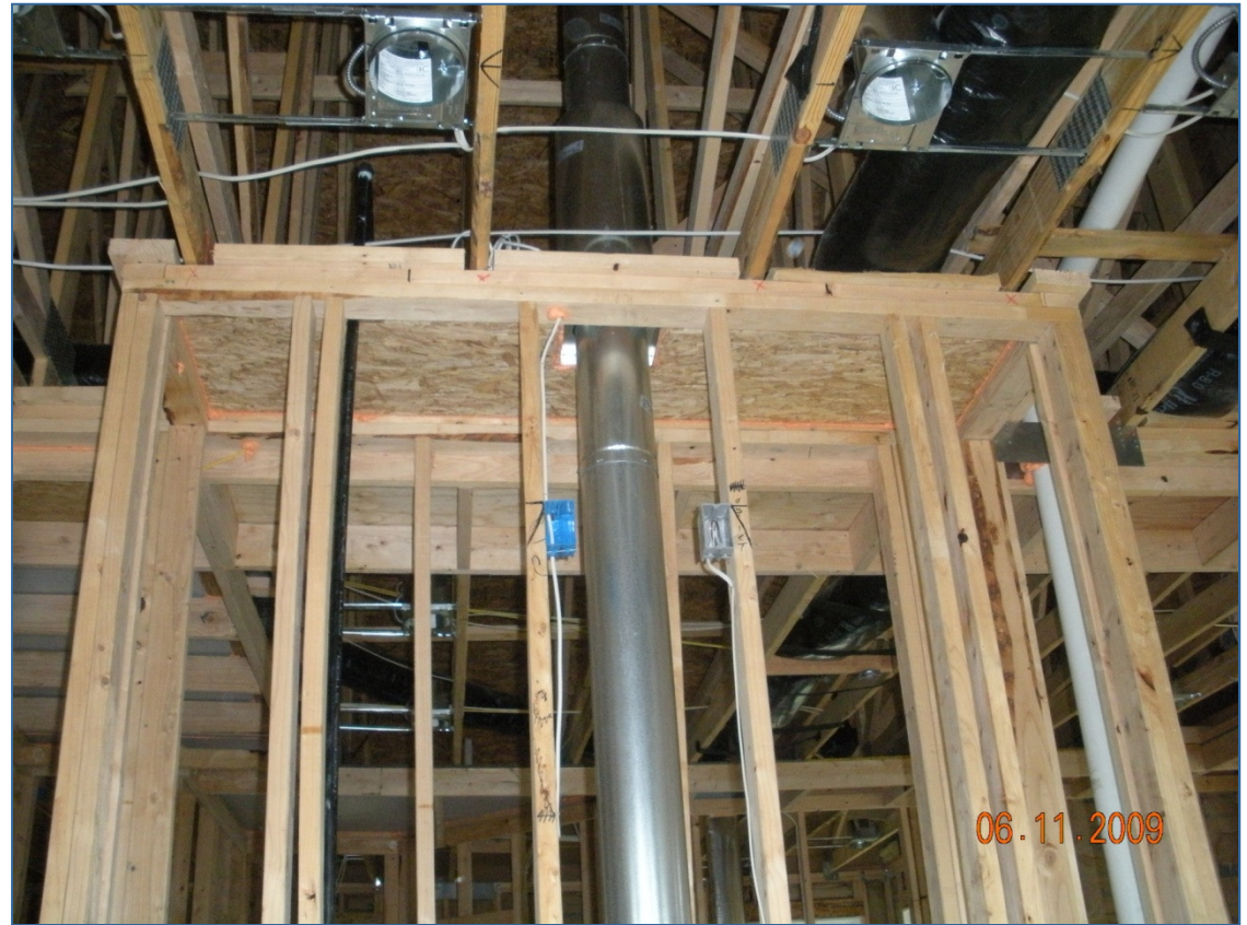
Sealed air barriers at fireplace framed cavity and coffered ceiling beyond
