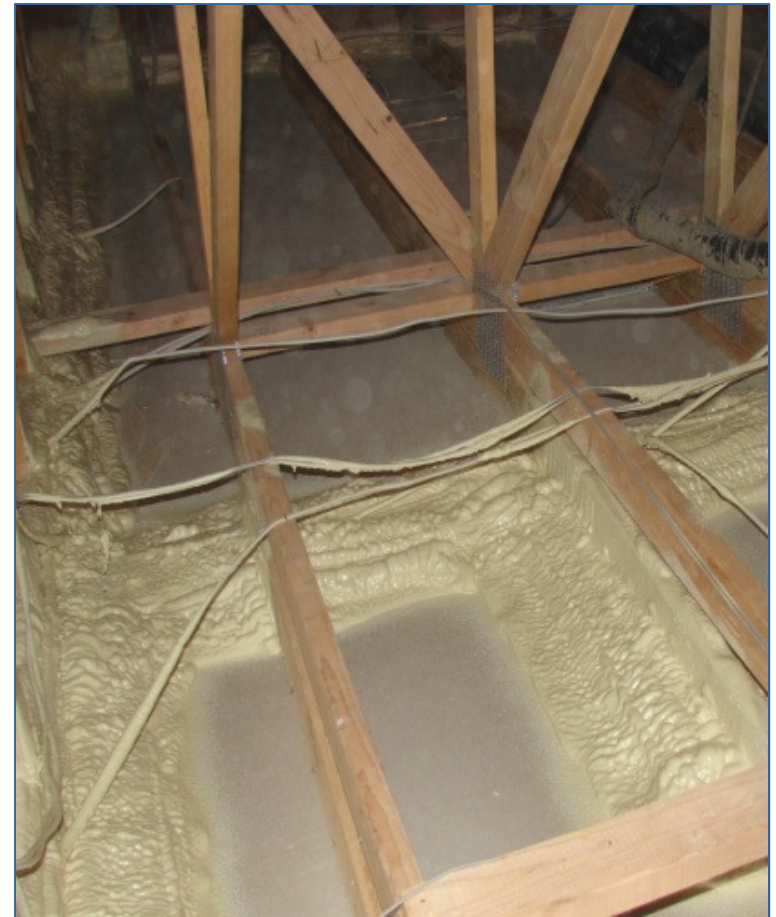
Top plates foamed from attic
