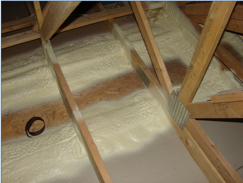
Sealed top plates and air barrier
