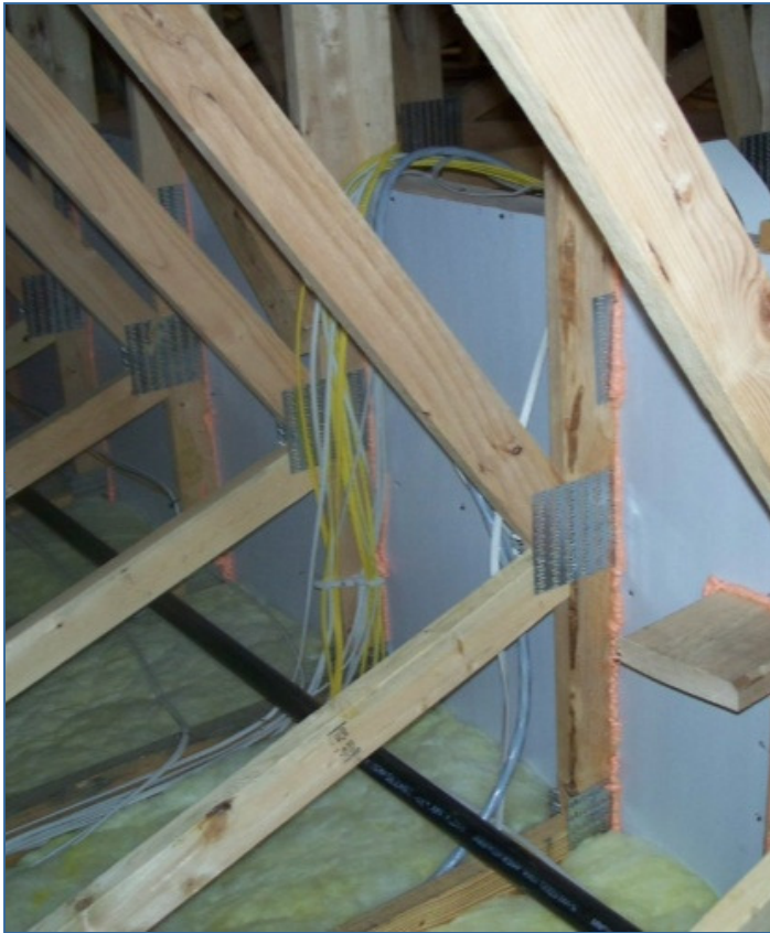
Sealed air barrier adjacent to garage knee wall
