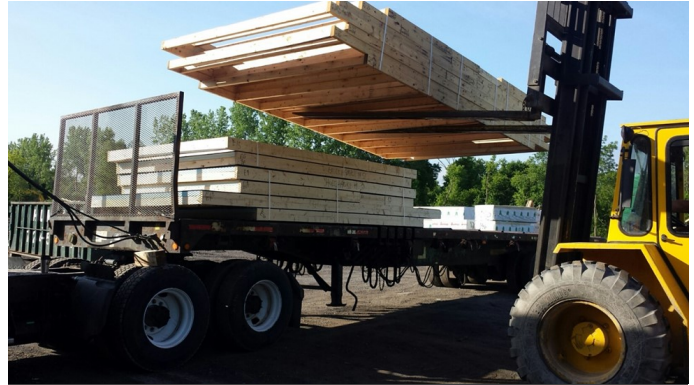
Figure 5. Factory Panelization Loading and shipping panelized wall sections from the factory.
