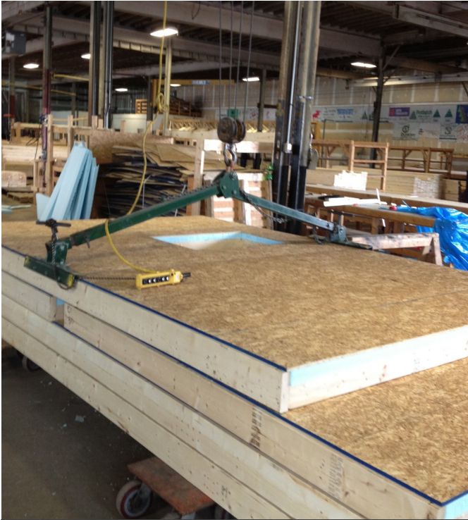
Figure 4. Factory Panelization Bundling and strapping panels.
