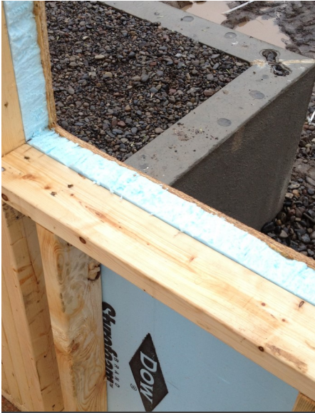
Figure 15. Openings Frame window openings with 2x4 lumber to maximize continuous insulation. Door openings for sliders can use full-depth framing for stability.
