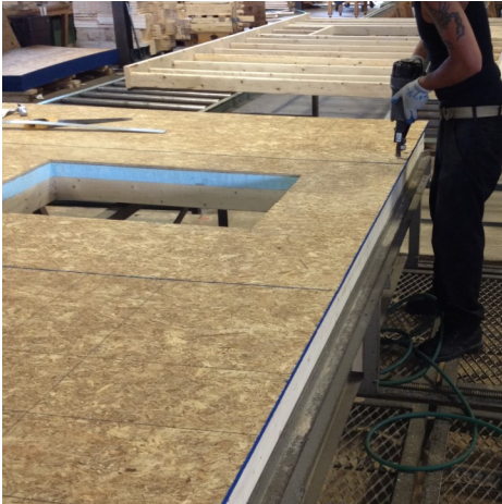
Figure 12. EP&B Wall Factory Fabrication
