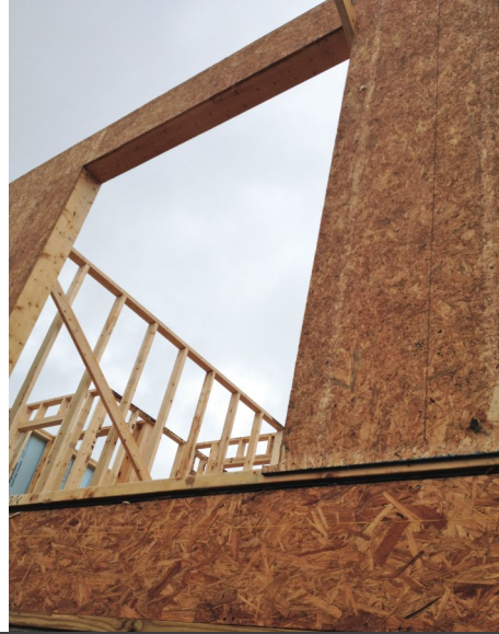
Figure 15. Openings Frame window openings with 2x4 lumber to maximize continuous insulation. Door openings for sliders can use full-depth framing for stability.
