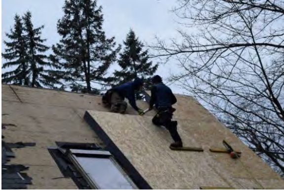
Figure 44. Retrofit panel installation on back of main roof
