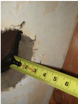
Figure 8. Michigan main house existing fiberboard roof deck/ceiling
