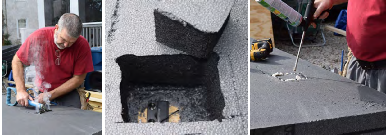
Figure 37. Sensor installation within retrofit panels
