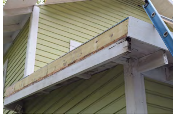
Figure 34. Polyvinyl chloride trim board was installed over the curbs
