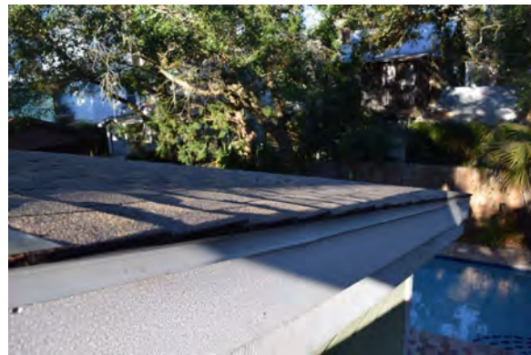
Figure 35. Ventilation mat and shingles on one-story roof
