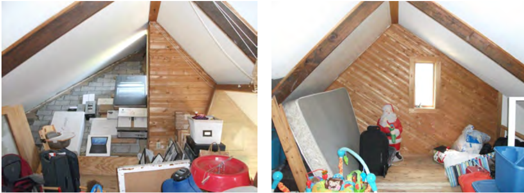
Figure 19. Michigan addition roof (Rafters shown are decorative.)
