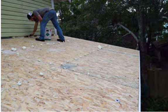
Figure 33. Retrofit panels sealed at panel-to-panel edges
