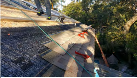
Figure 41. Ventilation mat and shingle installation
