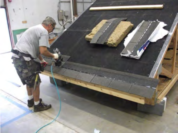
Figure 11. Installation of shingles
