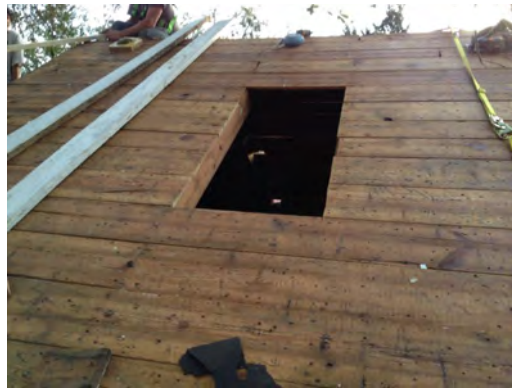
Figure 25. Construction access to attic at roof deck
