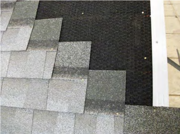
Figure 12. Installation of shingles and ridge vent
