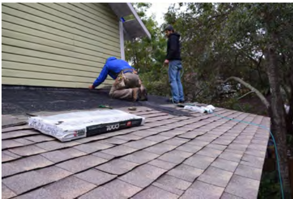
Figure 35. Ventilation mat and shingles on one-story roof
