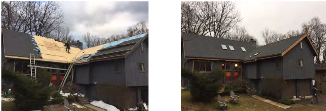
Figure 49. Installation progress and installation complete
