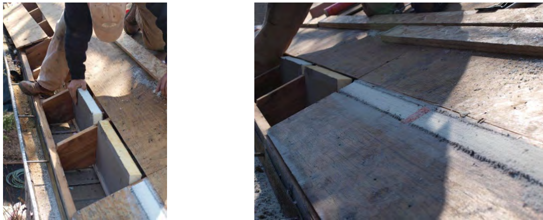
Figure 23. Example eave insulation method
