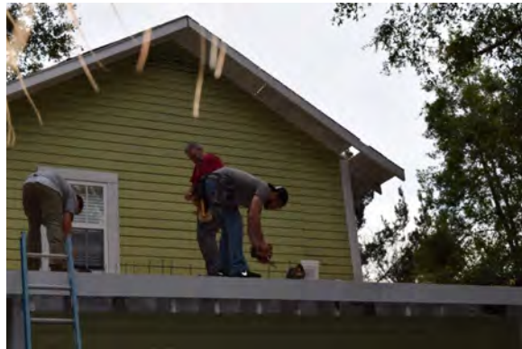
Figure 32. Panels were screwed into rafters
