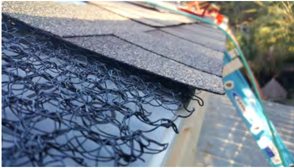
Figure 41. Ventilation mat and shingle installation
