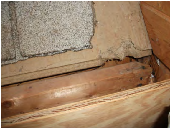
Figure 8. Michigan main house existing fiberboard roof deck/ceiling
