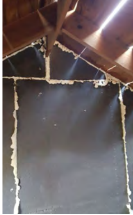
Figure 27. Rigid foam insulation at attic gable walls
