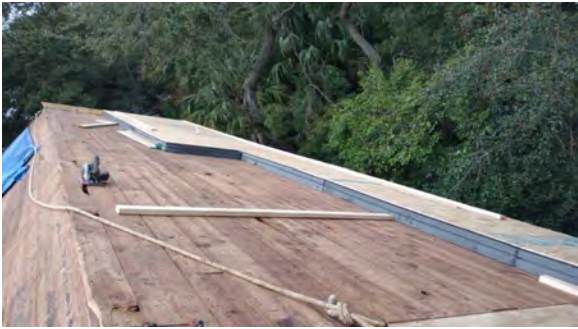
Figure 40. Panel installation progress on the second-story roof
