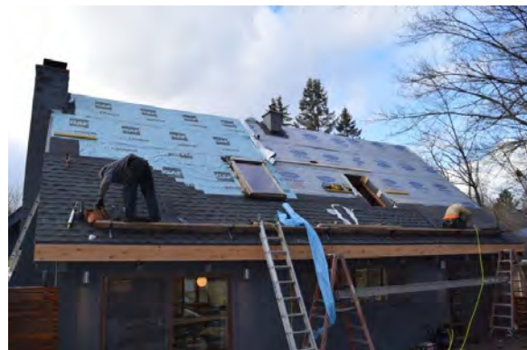
Figure 46. Skylights were removed and reinstalled after panels
