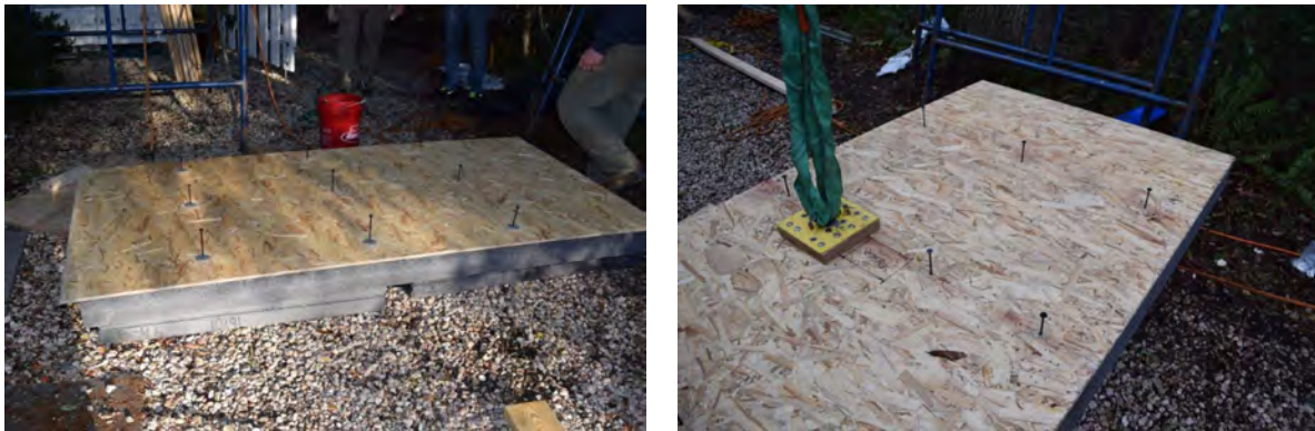
Figure 38. Pre-installed screws (Note the sensor location marked on the OSB next to the cleat.)
