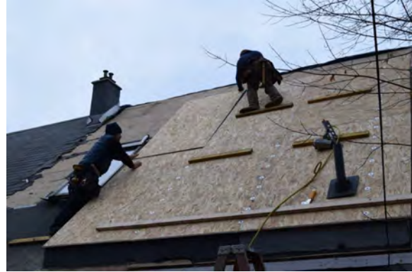
Figure 44. Retrofit panel installation on back of main roof
