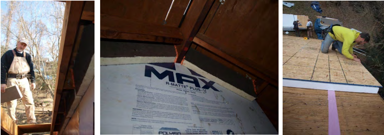
Figure 24. Example gable wall insulation method
