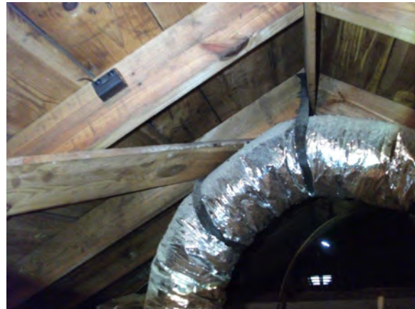
Figure 5. Georgia house eaves and roof framing with rafter sensor
