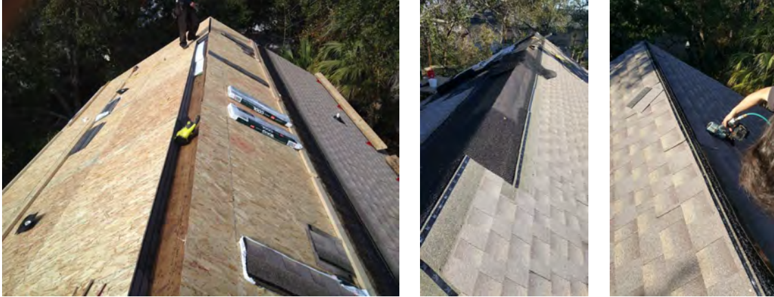
Figure 42. Panel and roofing during installation
