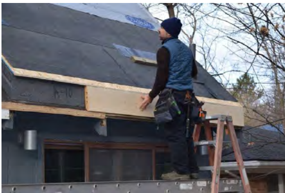
Figure 45. Nailing curbs installed after the retrofit panels
