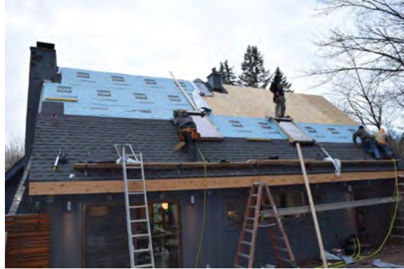
Figure 47. Roofing the back of the main roof
