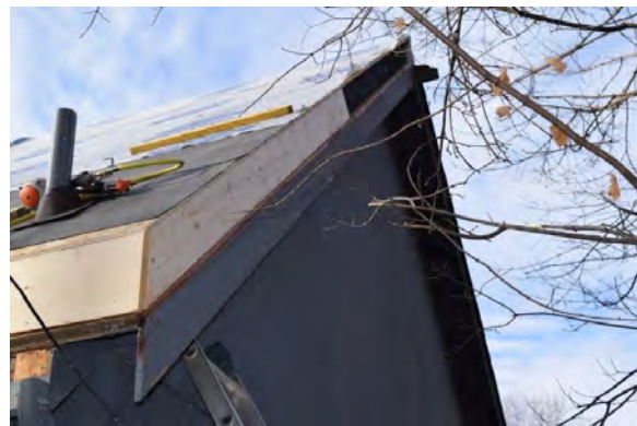
Figure 45. Nailing curbs installed after the retrofit panels
