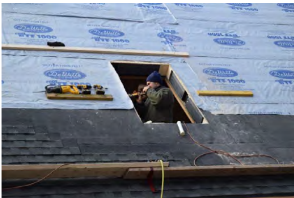
Figure 46. Skylights were removed and reinstalled after panels
