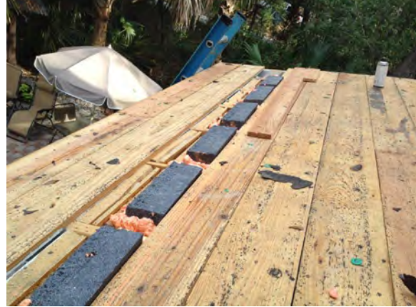
Figure 28. Rigid foam insulation at eaves
