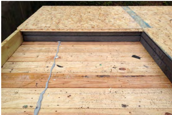
Figure 31. Oriented strand board surface spline and sealant at deck above rake wall
