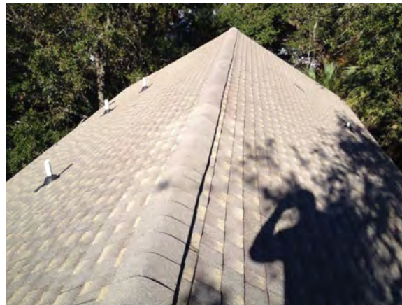
Figure 43. Second-story roof complete
