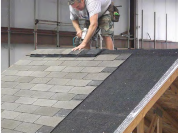
Figure 12. Installation of shingles and ridge vent
