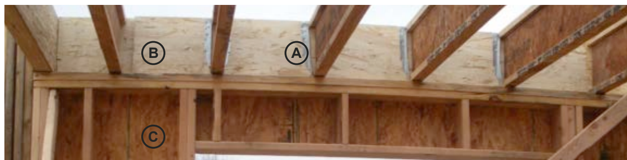
Rim header installation is similar to common floor joist to girder installation
