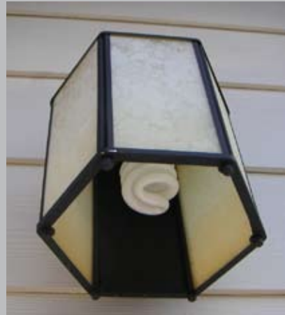
CFL in exterior light fixture Yavapai College, Residential Building Technology Program, 2007 EVHA Gold Winner
