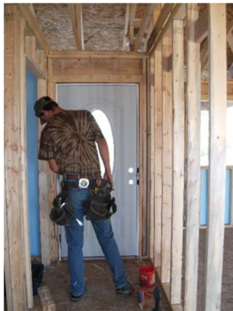
Exterior doors need 6-in. jambs to match the wall width of a 2x4/2x6 EP&B wall.
