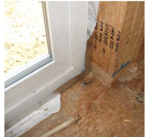
Sliding door installed in opening.
