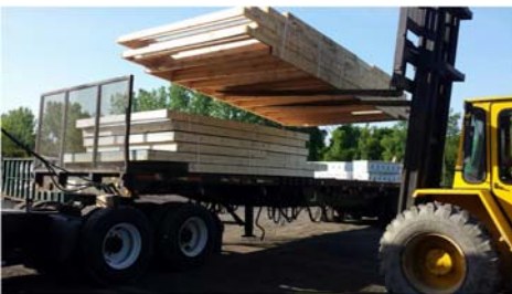
Factory Panelization —Loading and shipping panelized wall sections from the factory.
