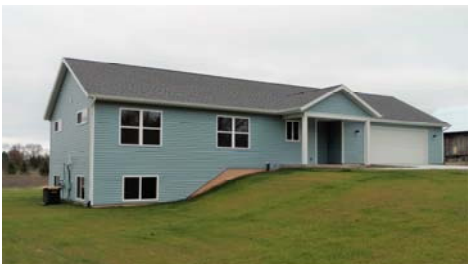
A completed EP&B demonstration home in Grand Rapids, Michigan.
