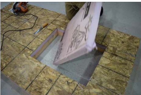
Remove the foam from the opening.
