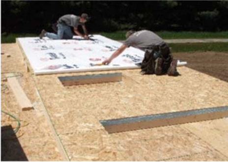
Attach WRB before wall erection to save time and effort. Use cap nails or wide staples per manufacturer's requirements.
