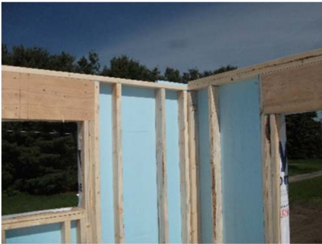
Fill in the EP&B components at the outside corners of the short wall—OSB.
