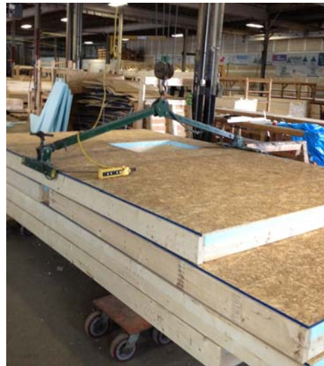
Factory Panelization —Bundling and strapping panels.
