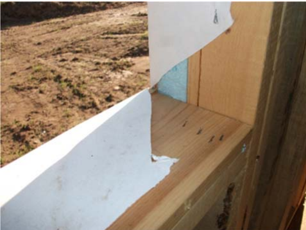
Window opening, WRB folded back, 1x6 sill plate added (not required).
