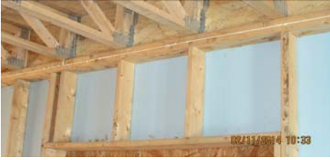
Double Rim Beam as header; note joist hangers and caulk sealing.
