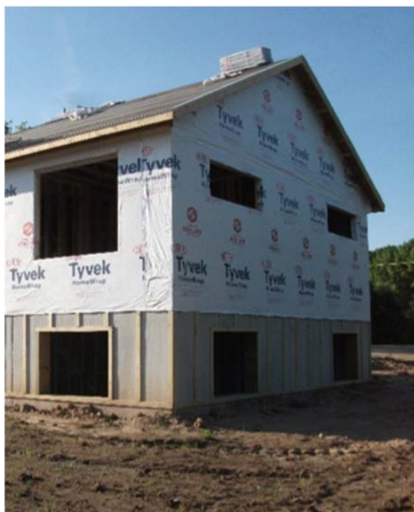
Apply WRB and siding with standard methods.
