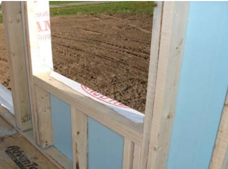
1x6 sill added (not required).
