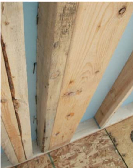
If nails missed the stud, re-nail from outside.
