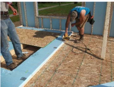
At outside corners, plan temporary gaps in the foam and OSB to leave knuckle room for erection and connection. The last sections of foam and OSB can then be added from the exterior side of the building. Ensure that foam and OSB joints do not land at the same stud.
