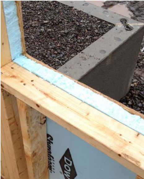
Frame window openings with 2x4 lumber to maximize c.i.
