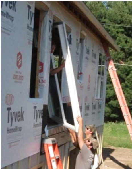
Install windows and doors only after the opening has been properly detailed.
