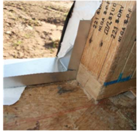
Apron and stainless steel pan at sliding door opening, leading to elevated deck on the north side of the house.
