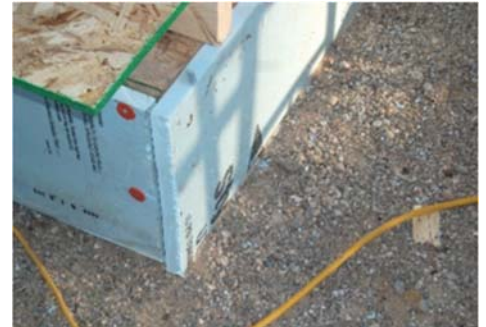
Ensure a complete thermal break.
