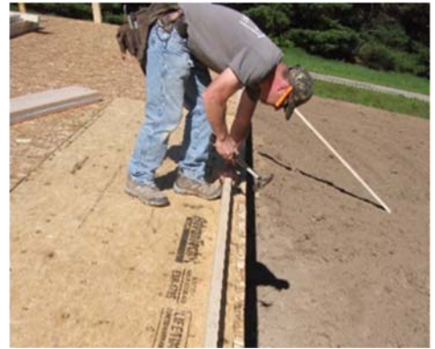
Temporarily nail bottom plate to deck.
