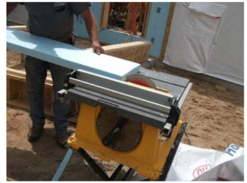
A table saw trims 2-in. rigid foam cleanly, with little waste or debris.
