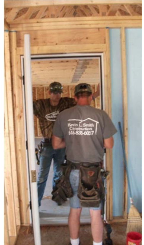
Plumbing the door.
