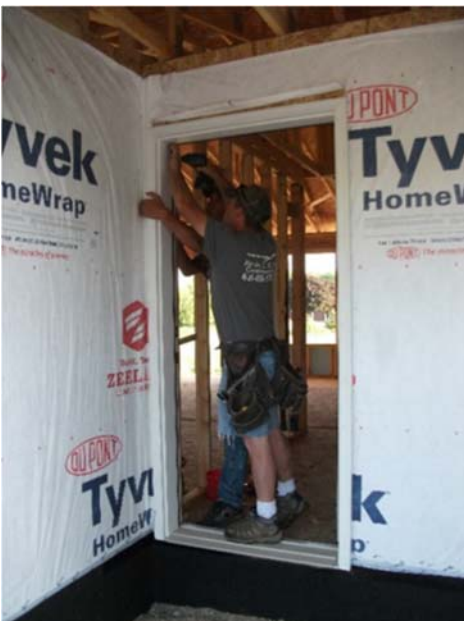
Nailing the door frame.
