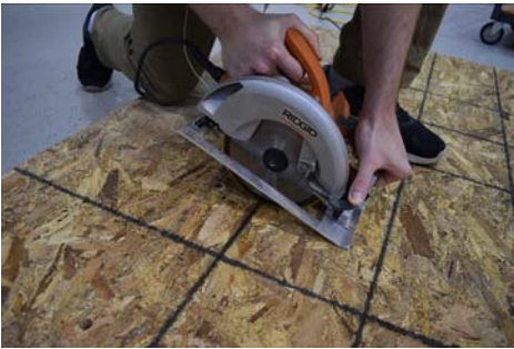
Sink the circular saw to catch the first drill hole. Do not overcut at corners.
