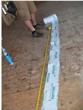
Flexible, self-adhered pan flashing tape, cut to length.
