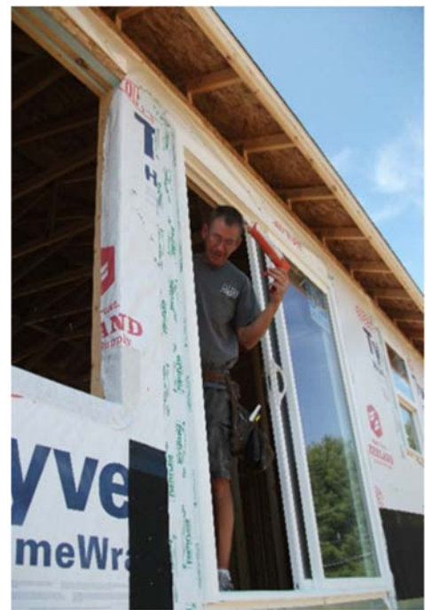
Caulk or seal with WRB tape all new penetrations through flashing.
