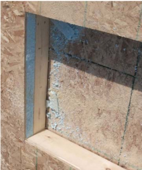
1x6 sills may be added for convenience but are not necessary.
