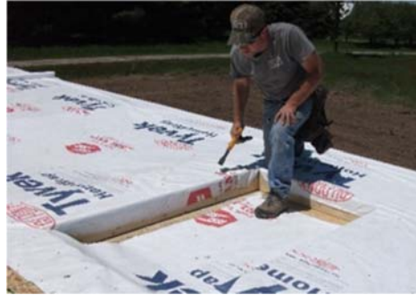
Cut window openings. See window installation and detailing guidance on page 22.
