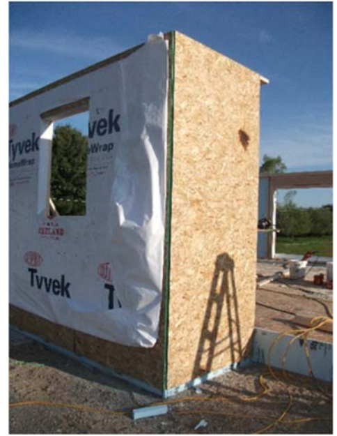
Plan outside corners carefully to anticipate the layering of rigid foam, OSB, and WRB, and a bead of caulk or spray foam for air-sealing.
