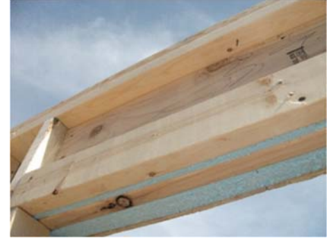
Single header, with 2x4 nailer.
