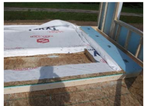
At outside corners, plan temporary gaps in the foam and OSB to leave knuckle room for erection and connection. The last sections of foam and OSB can then be added from the exterior side of the building. Ensure that foam and OSB joints do not land at the same stud.
