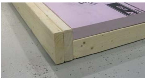
The final recommended EP&B configuration uses two extended top plates, in addition to the extended bottom plate.
