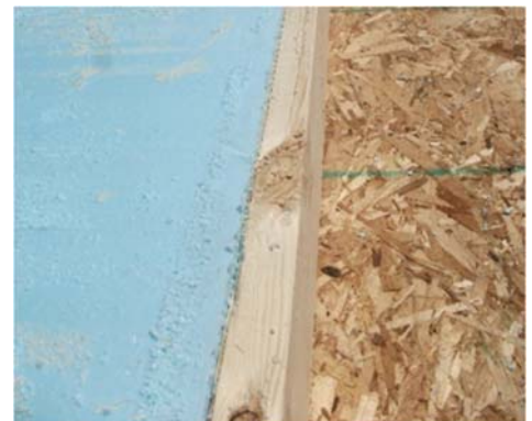
Adjust the height of the circular saw blade to protect the framing.
