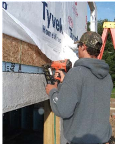
Where possible, re-nail before fully attaching the WRB.
