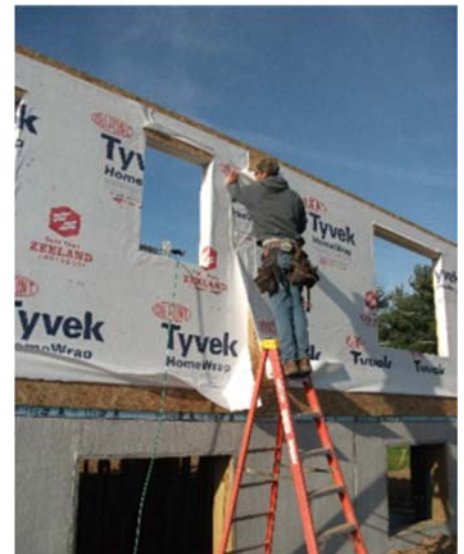
If it's necessary to nail through the WRB, seal each nail head with tape or caulk.
