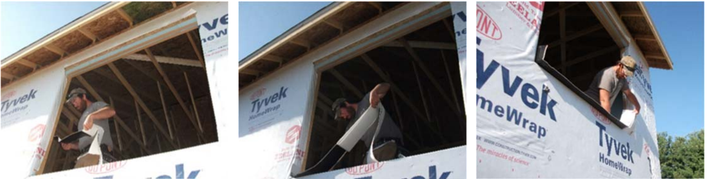
Apply flexible, self-adhered pan flashing, extending several inches up the jamb on each side. Smooth out all wrinkles.
