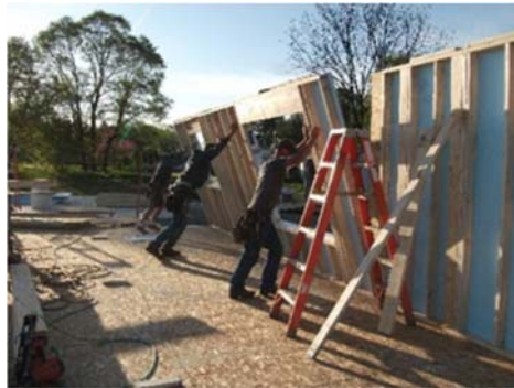
Plan the layering of foam and OSB so vertical material joints between adjacent panels occur at different studs.
