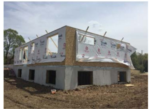
Fill in the EP&B components at the outside corners of the short wall—OSB.
