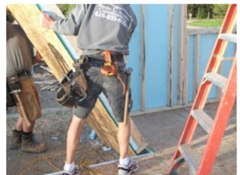
It is not possible to add foam or caulk once an exterior corner is in place, unless the OSB is added after erection.
