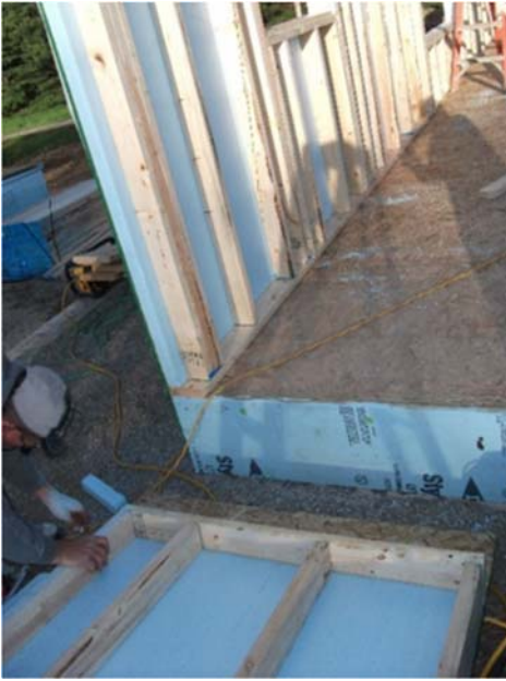
Plan outside corners carefully to anticipate the layering of rigid foam, OSB, and WRB, and a bead of caulk or spray foam for air-sealing.
