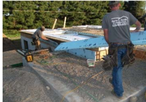
Tack c.i. rigid foam to rim band.
