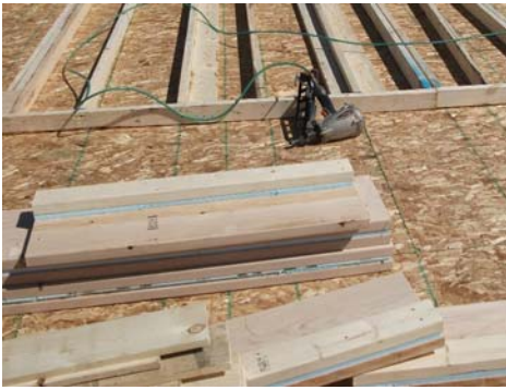
Double headers have a 1-in. foam sandwich; single headers have a 2x4 nailer added at bottom for attaching window trim.
