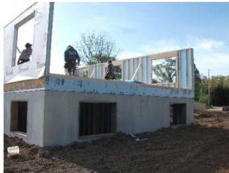
Plan short, connecting end walls carefully to maintain an uninterrupted layer of rigid foam across outside corners. Remember to apply a bead of caulk prior to tipping up, and follow with caulk if necessary to ensure an air-seal.
