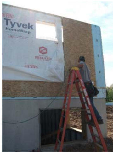
Fill in the EP&B components at the outside corners of the short wall—OSB.
