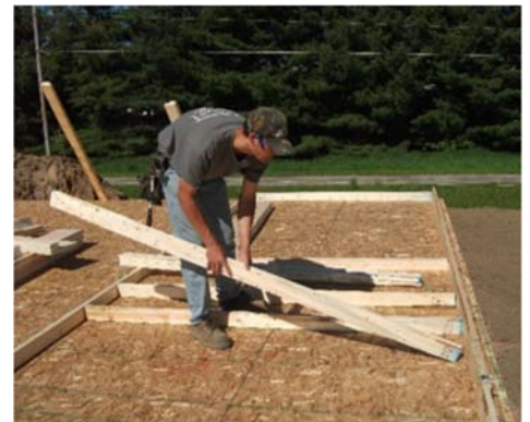
Lay out studs and framing lumber according to plan. Remember that in the final recommended EP&B configuration, all three plates should be the same dimension.
