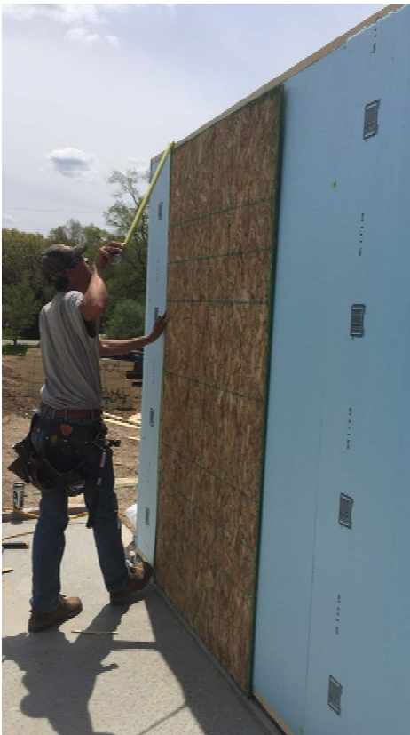
OSB sheathing must always be oriented vertically, for structural bracing.
