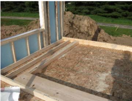
Plan short, connecting end walls carefully to maintain an uninterrupted layer of rigid foam across outside corners. Remember to apply a bead of caulk prior to tipping up, and follow with caulk if necessary to ensure an air-seal.
