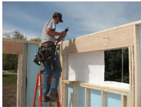
Final detailing of outside corner connections.
