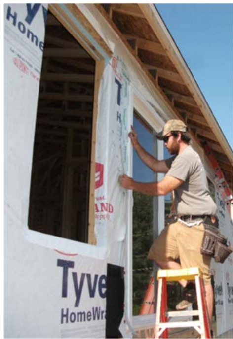
Smooth wrinkles and press out air pockets to avoid imperfections that can trap water.
