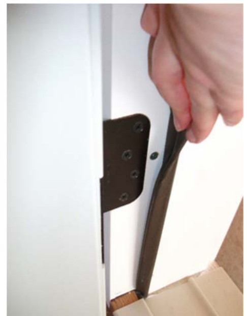
The factory-drilled securement jamb holes match up with the framing of an EP&B wall.
