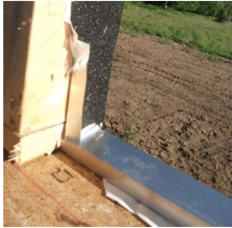
Apron and stainless steel pan at sliding door opening, leading to elevated deck on the north side of the house.
