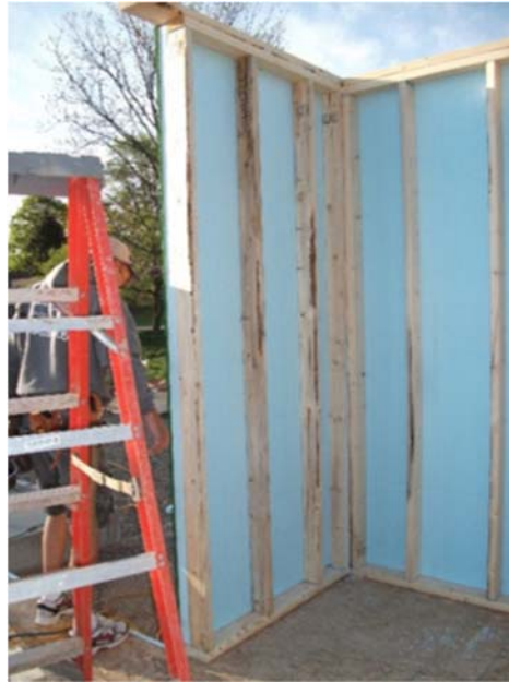
Plan outside corners carefully to anticipate the layering of rigid foam, OSB, and WRB, and a bead of caulk or spray foam for air-sealing.
