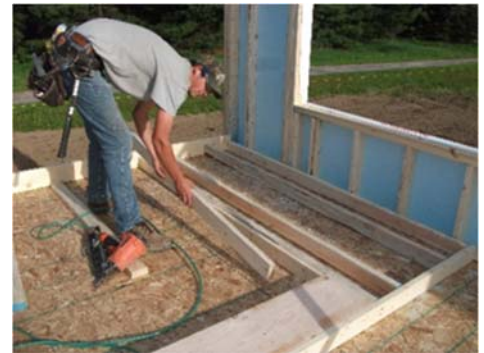
Plan short, connecting end walls carefully to maintain an uninterrupted layer of rigid foam across outside corners. Remember to apply a bead of caulk prior to tipping up, and follow with caulk if necessary to ensure an air-seal.
