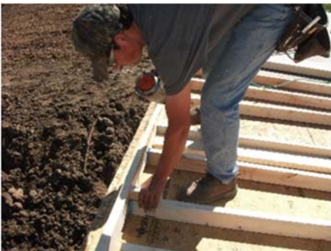
Use the spacer when end-nailing studs to measure the gap for the foam layer.
