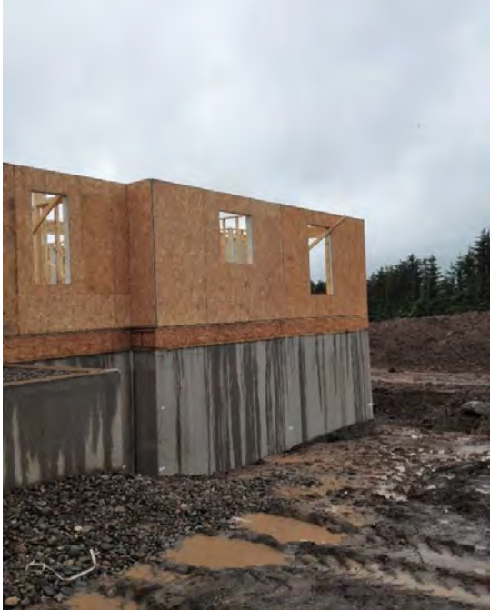
Figure 21. EP&B Panels Tipped up and Braced
