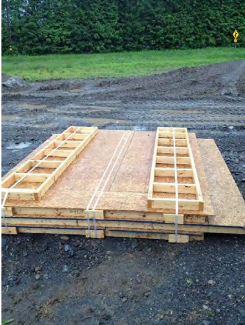
Figure 20. Wall Panels Unloaded on Site
