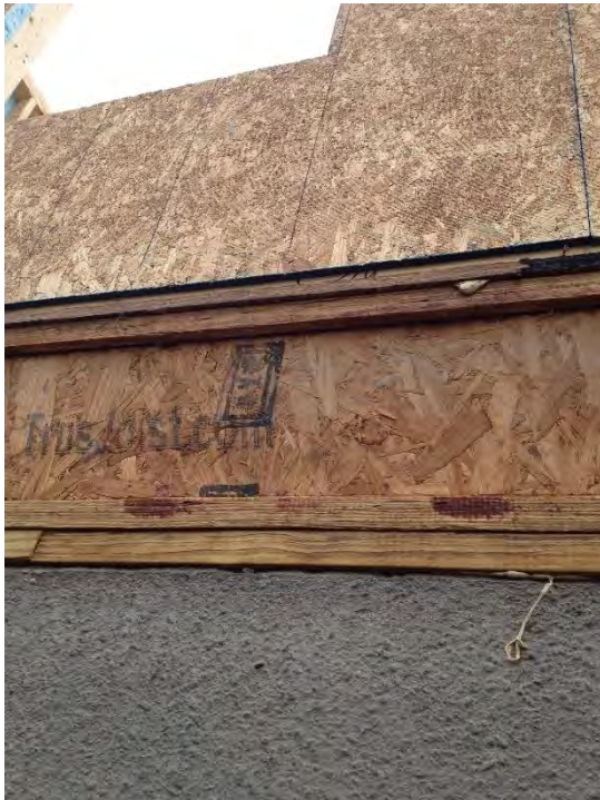
Figure 22. Engineered Rim
