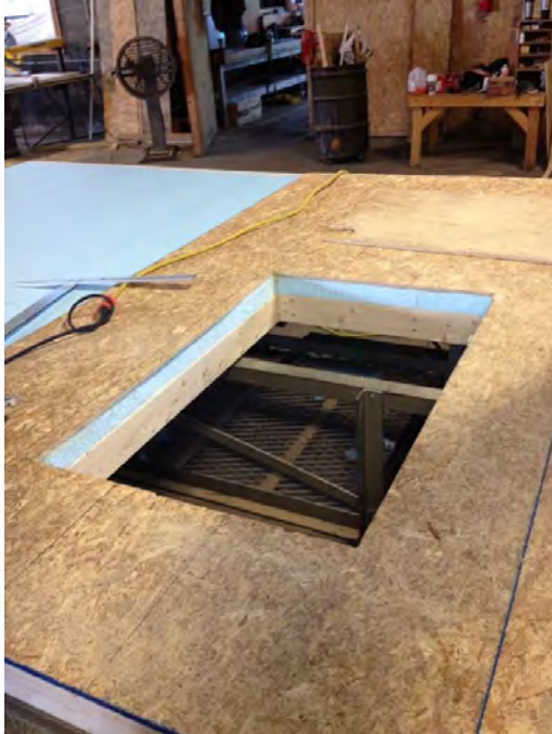
Figure 13. A Wall Panel with a Window Opening
