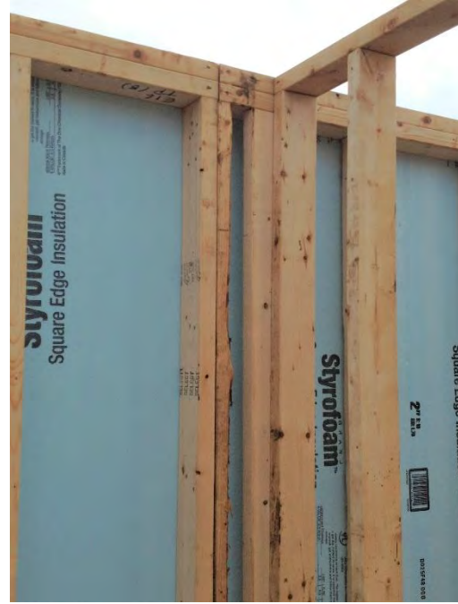
Figure 28. Interior Partition Wall Connection
