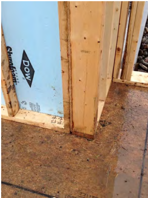
Figure 29. Outside Corner Connection
