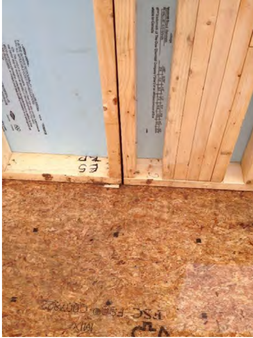
Figure 27. Connection Between EP&B Wall Panels
