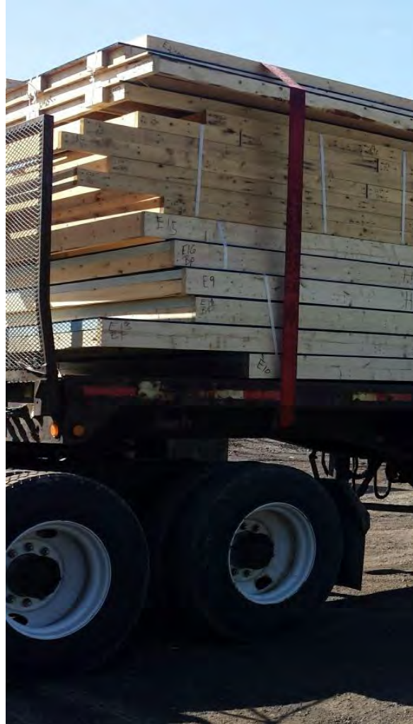
Figure 18. EP&B Panels Strapped onto Trailer for Transport to the Project Site
