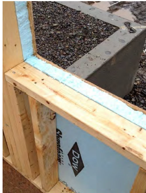
Figure 26. Typical EP&B Window Opening
