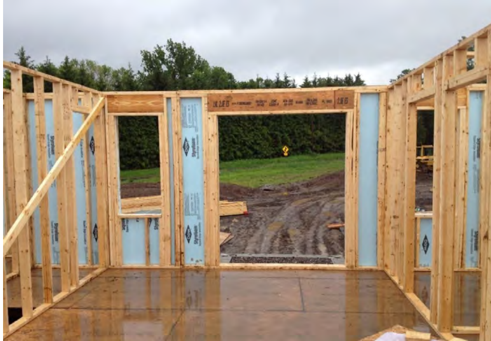
Figure 24. EP&B Wall Panels Braced in Place
