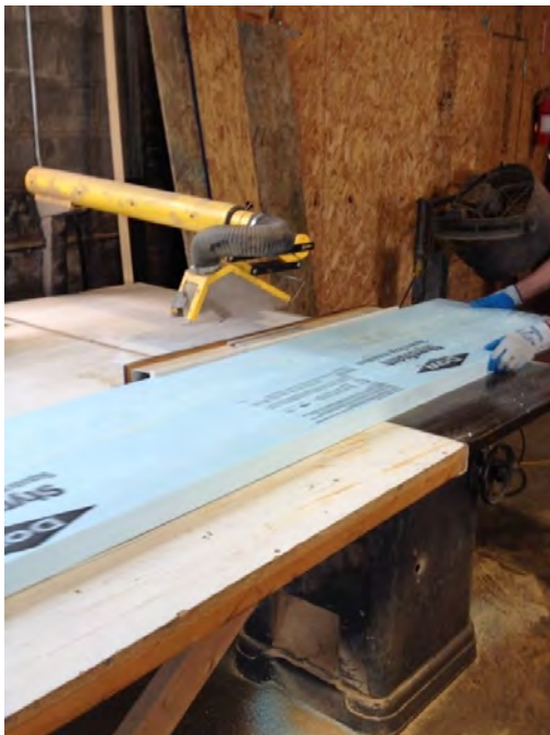
Figure 15. Cutting XPS on a Table Saw
