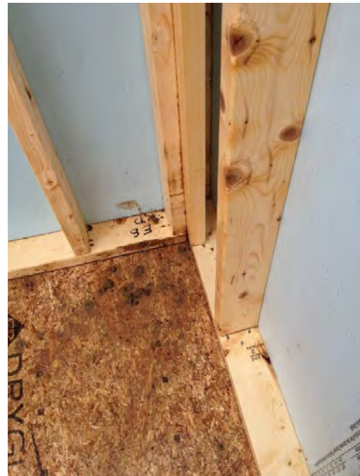
Figure 30. Inside Corner Connection
