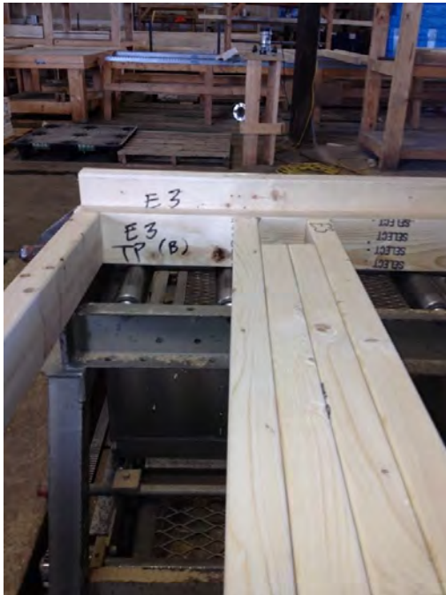
Figure 11. Studs Nailed to Bottom Plate, leaving 2-in. Gap for Foam
