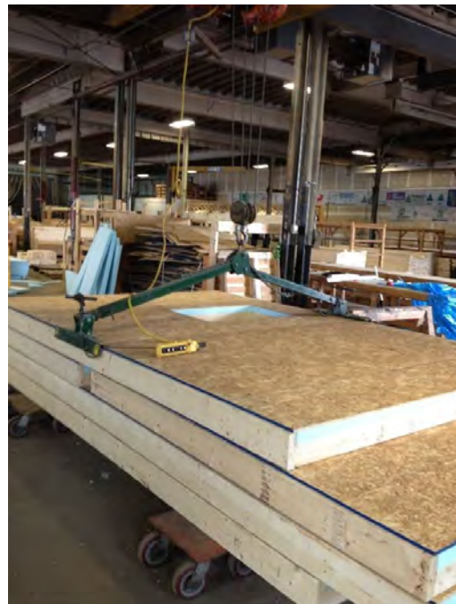
Figure 16. Grouping Finished Wall Panels for Bundling and Shipping
