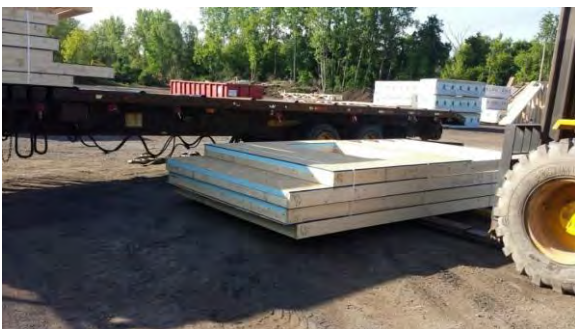
Figure 19. Loading EP&B Wall Panels onto Flatbed Trailer
