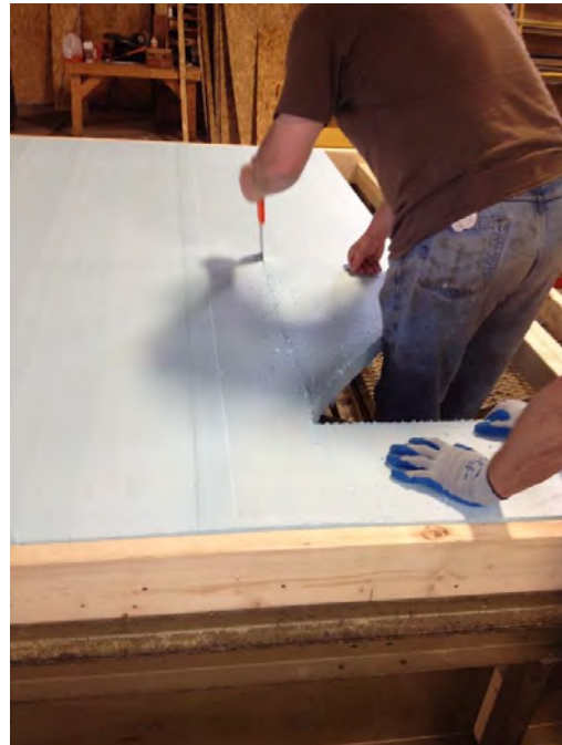
Figure 12. Using Hand Saw to Cut Foam for Windows
