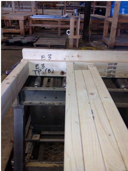
Figure 56. Studs nailed to bottom plate, with 2-in. gap for foam
