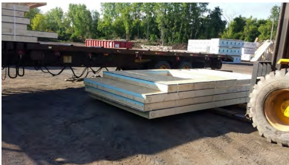
Figure 60. Loading EP&B wall panels for delivery
