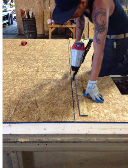
Figure 59. Using a guide to attach OSB to framing
