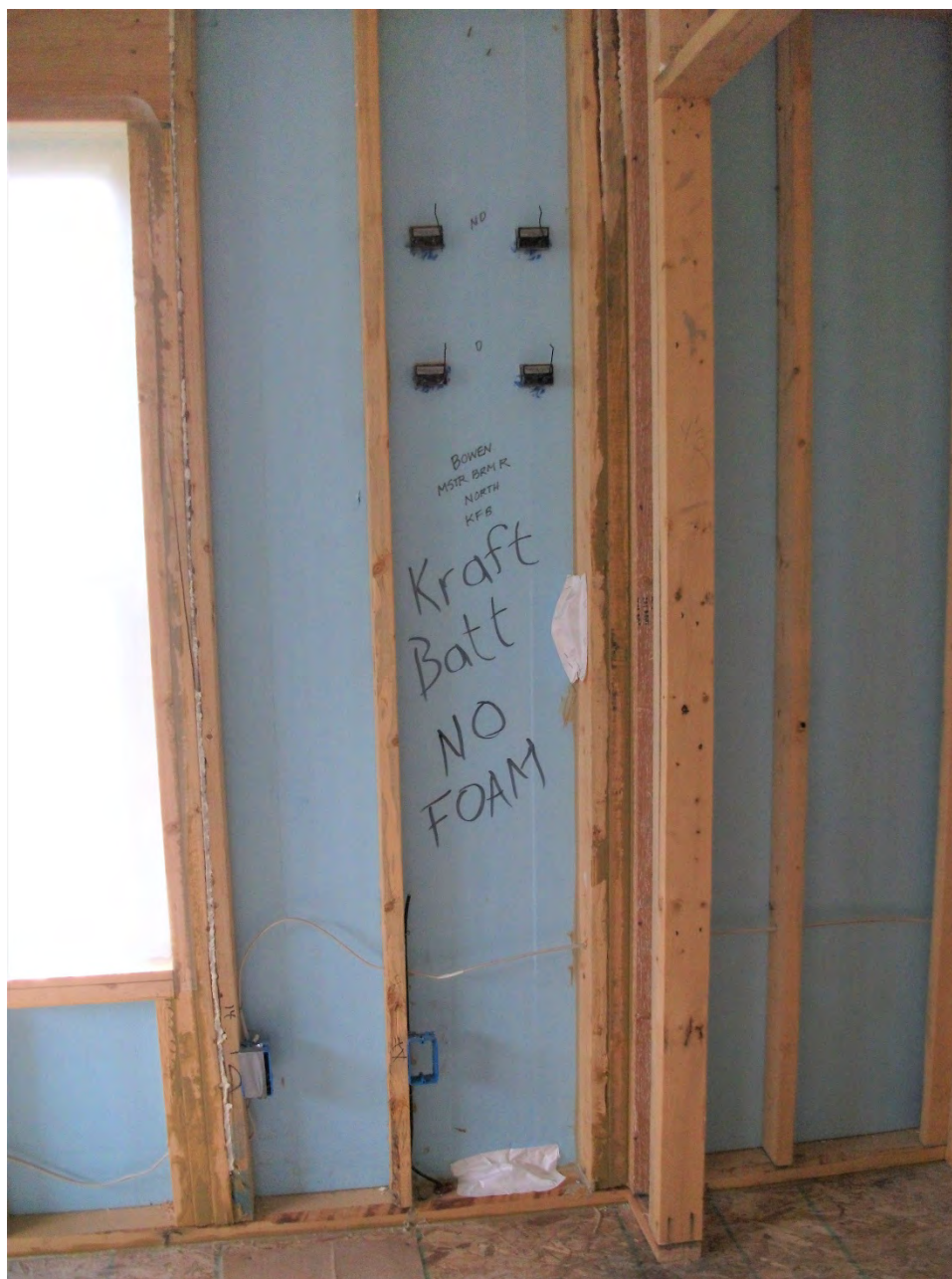
Figure 66. Bay containing outlier OSB sensor, House 1
