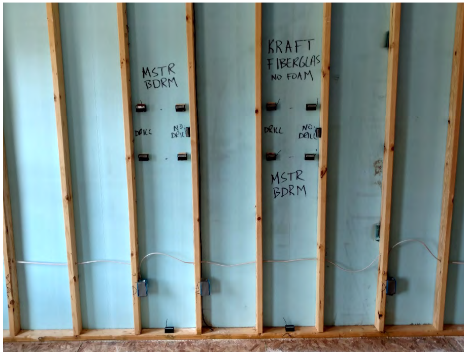
Figure 68. Wall containing outlier OSB sensor, House 2
