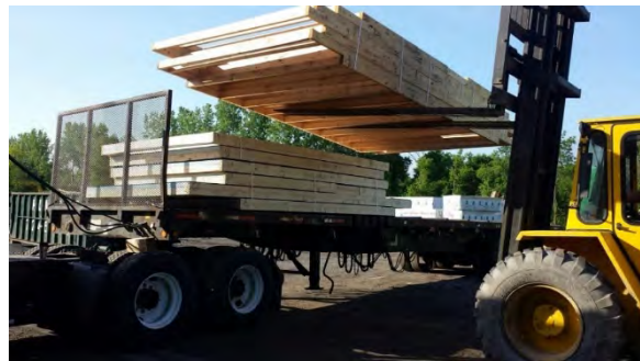
Figure 60. Loading EP&B wall panels for delivery
