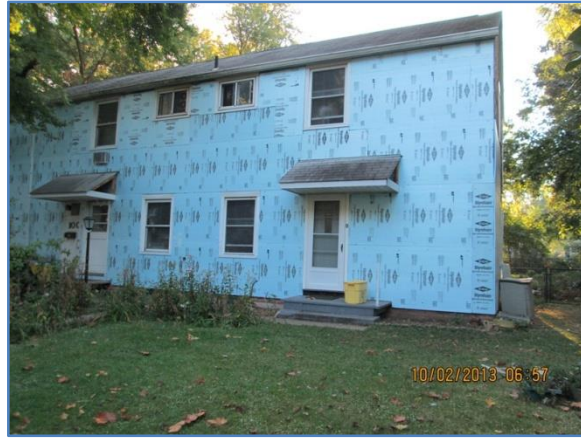
Figure 40. Foam Sheathing Installed
