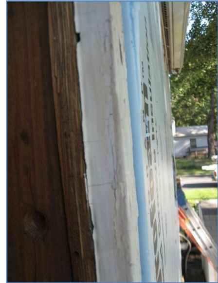
Figure 31. Foam Board Extends Beyond Original Window Trim
