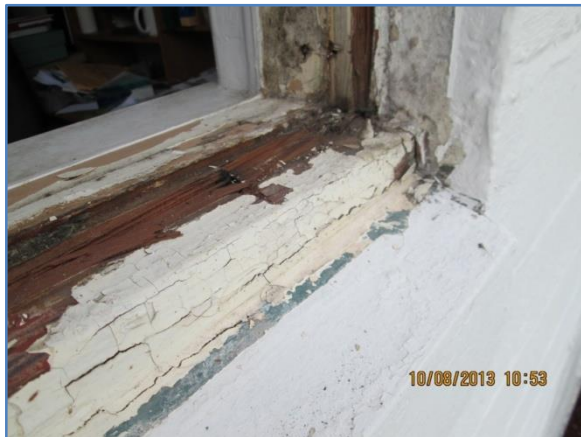
Figure 18. Window Rough Opening Prior to Window Install
