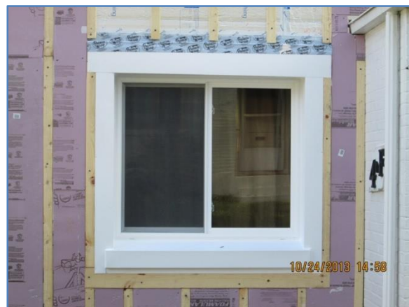
Figure 21. Window Flashing Integrated with Foam Insulation
