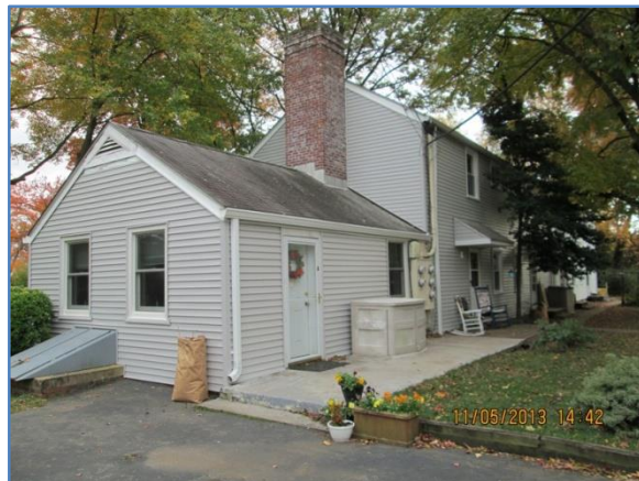
Figure 42. New Siding Installed Following Windows, Doors, Insulation, and WRB
