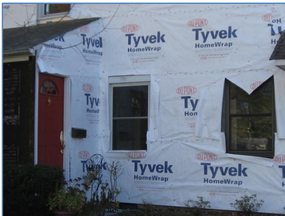
Figure 36. WRB Installed Over Foam Sheathing (not shown)
