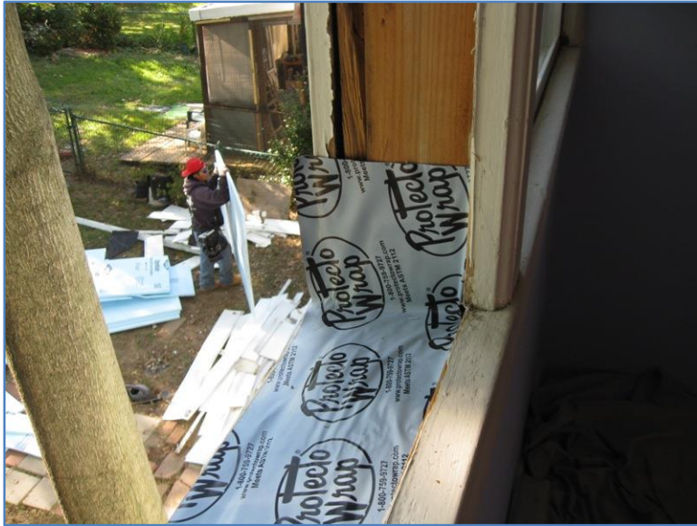
Figure 30. Window sill flashing on an FV unit
