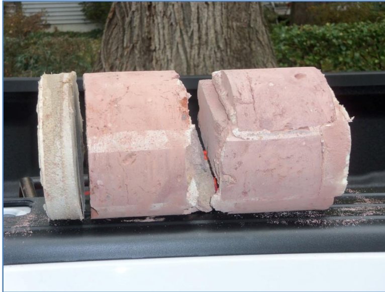
Figure 43. Core from Block Home for an Exhaust Fan
