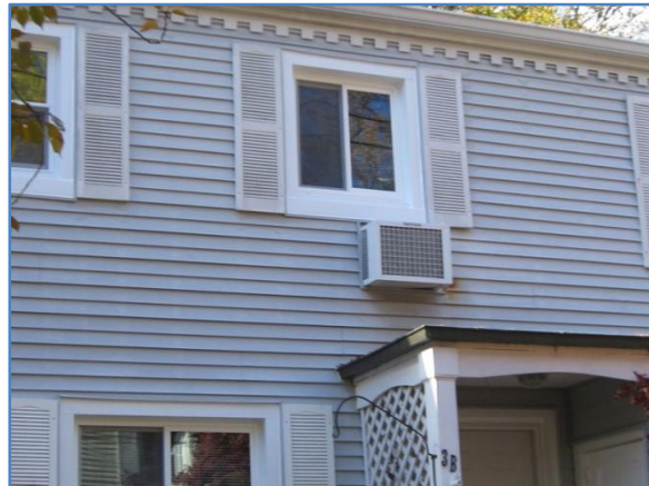
Figure 23. BV Building with New Windows and Trim
