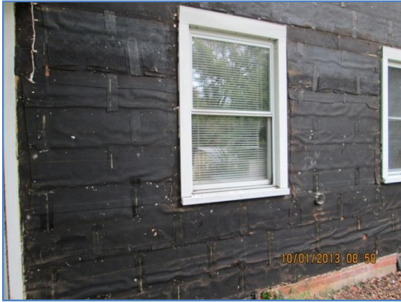
Figure 39. Original Building Paper on Frame Building
