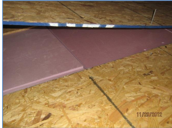
Figure 13. Wood Sheathing Installed Over the Foam Board to Maintain an Attic Storage Area
