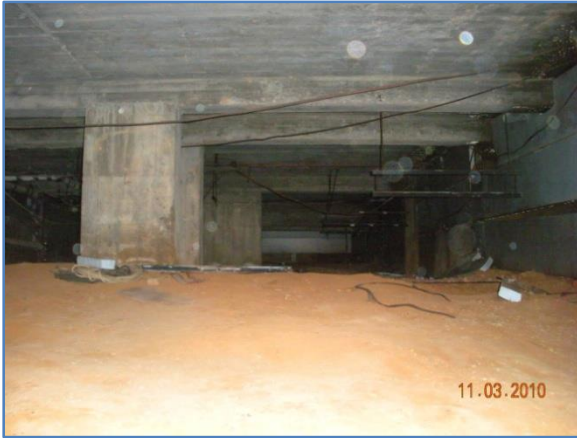
Figure 9. Block Building Crawlspace Prior to Upgrades
