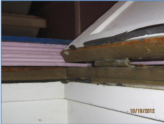
Figure 12. Foam Board at Attic Storage Area
