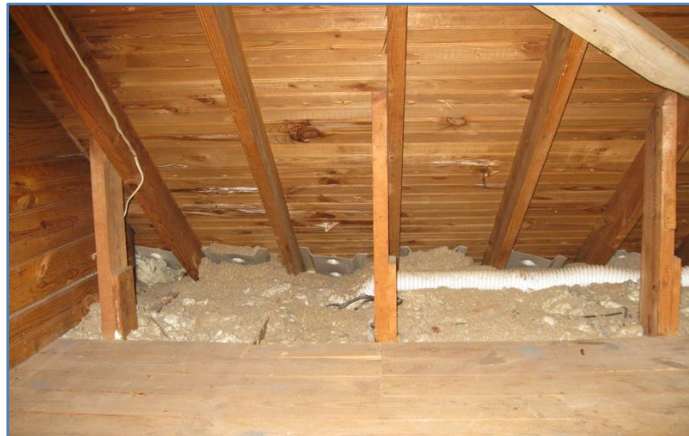
Figure 11. Typical Attic of the Wood Framed Buildings
