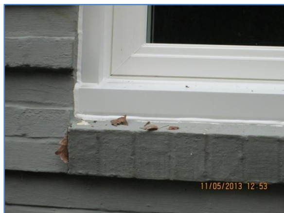
Figure 28. FB Replacement Window – Flashing and Caulking
