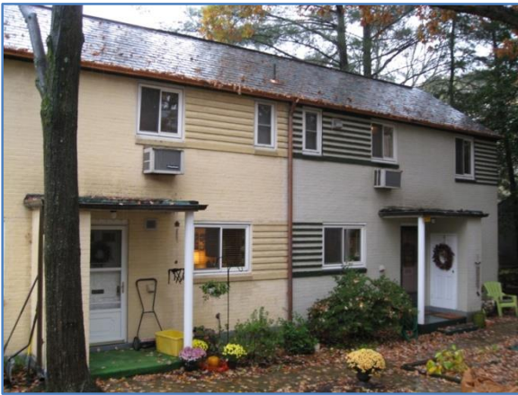
Figure 1. Frame-Brick Building (2 of 4 Homes in Set)
