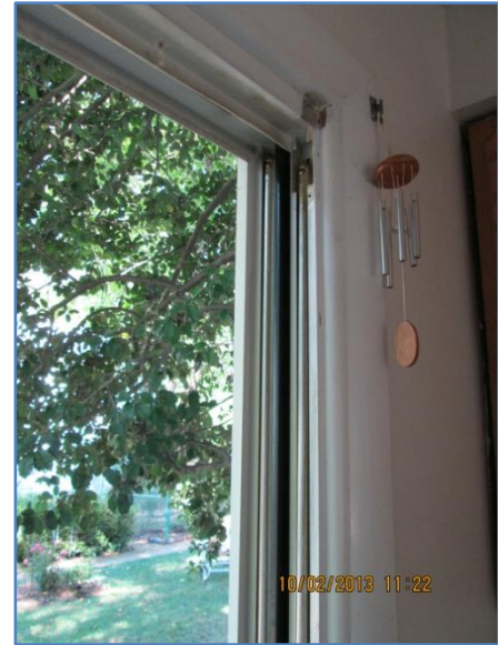
Figure 35. Replacement Window Installed and Flashed
