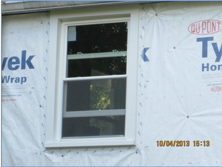
Figure 34. Additional Window Trim and Foam Sealing
