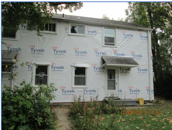
Figure 41. WRB Installed Over Foam Sheathing
