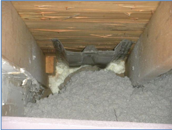
Figure 16. Exterior Top Plate Air Sealing
