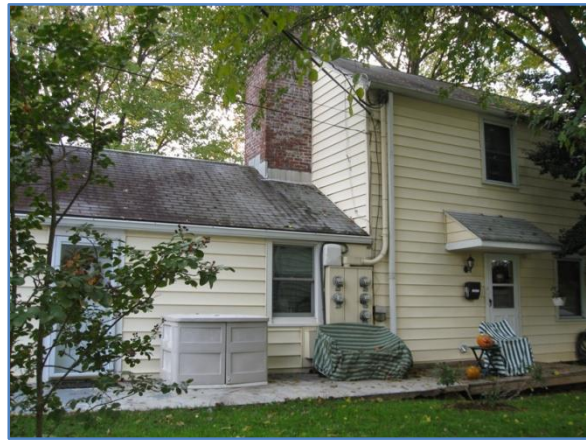
Figure 2. Frame-Vinyl Building (1st Home of 4 in Set)
