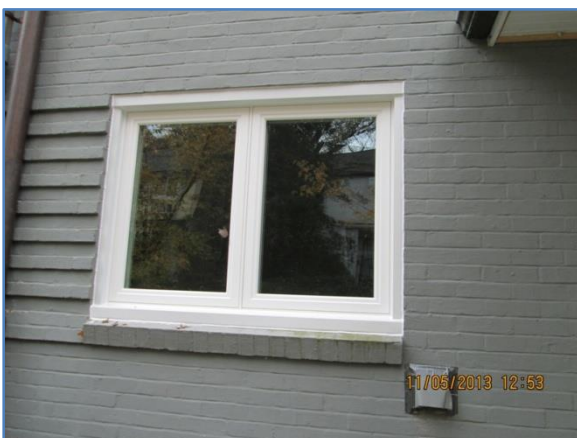
Figure 27. Replacement Window in FB Unit
