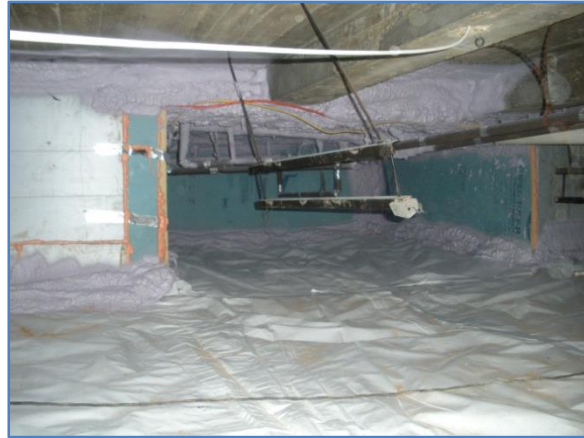
Figure 10. Building Crawlspace After Repair/Retrofits
