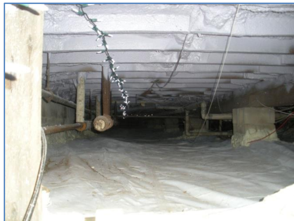
Figure 8. Frame-Vinyl Crawlspace After Upgrades
