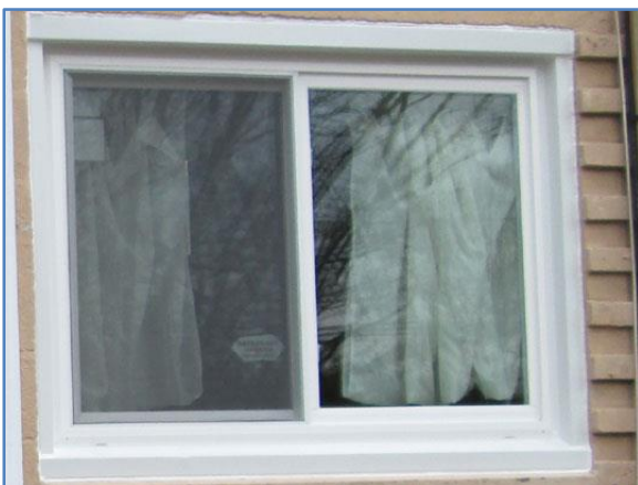
Figure 20. Window Trim Installed to the Block Rough Opening and Caulked
