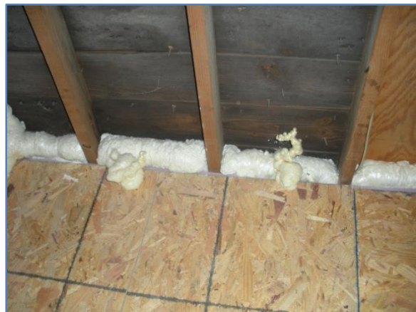
Figure 15. Gable End Wall Air Sealing
