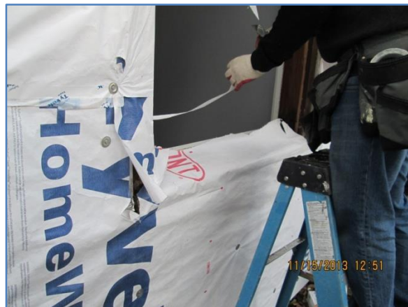
Figure 37. WRB Wrapped into Window Opening
