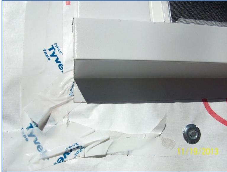
Figure 38. Window Trim Flashing Integrated with WRB
