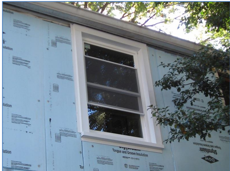
Figure 33. Replacement Window Installed and Flashed
