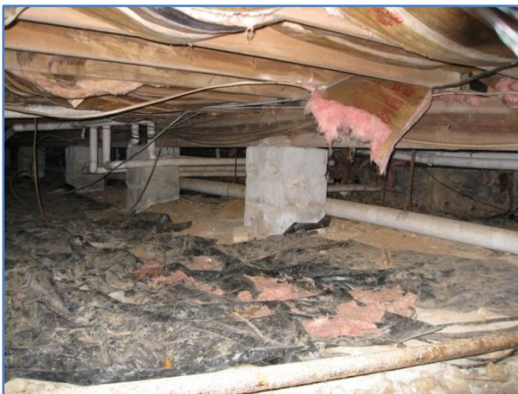
Figure 7. Frame-Vinyl Building Crawlspace Prior to Upgrades
