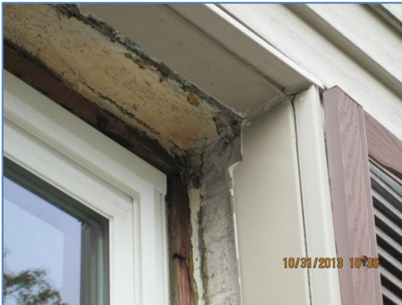
Figure 22. Replacement Window Installed in a BV Unit
