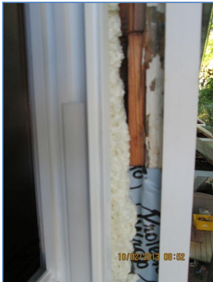
Figure 32. Additional Window Trim and Foam Sealing
