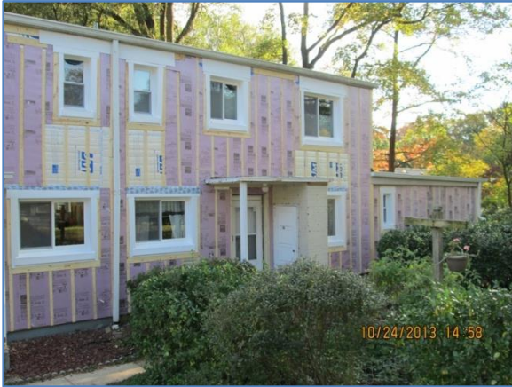
Figure 25. Block Building with Exterior Insulation Installed
