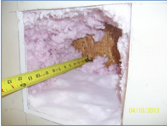
Figure 53. Insulation Removed from R-46 Wall for Observation
