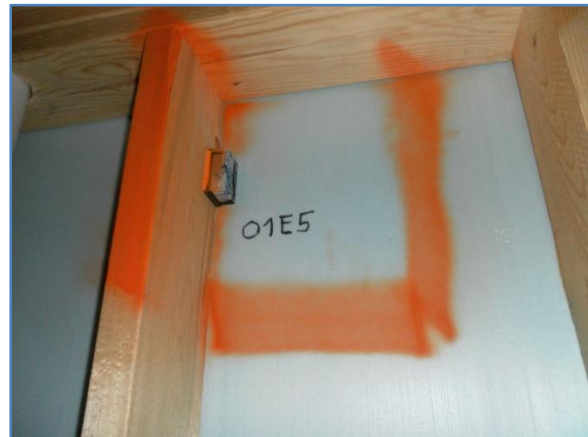
Figure 6. Sensor Installed in Lumber in Cavity With Only Foam Sheathing
