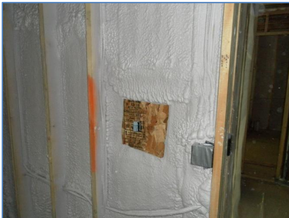
Figure 5. Sensor After Foam Flash and Before Insulation
