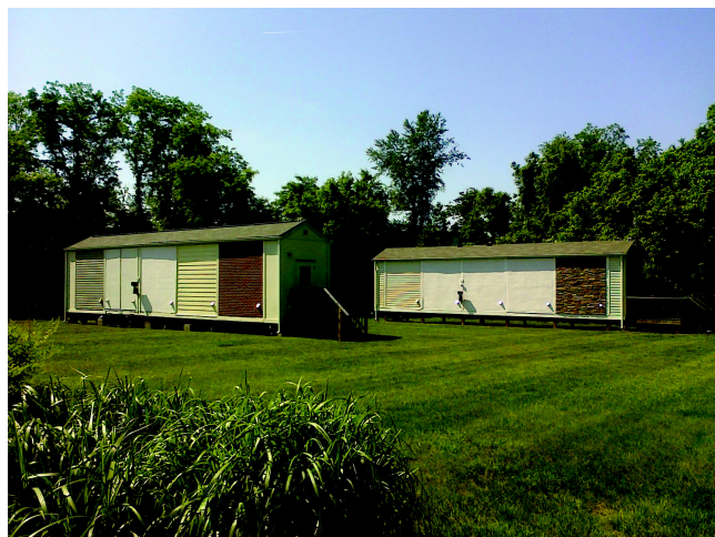
Figure 2 Test buildings 1 (right) and 2 (left).
