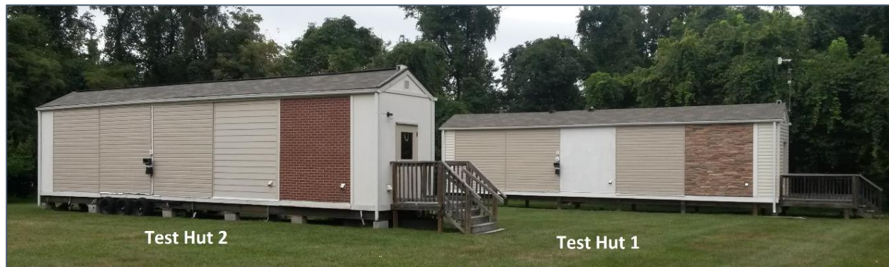
Figure 1. South Facing Walls of Test Structures 1 (right) and 2 (left)
