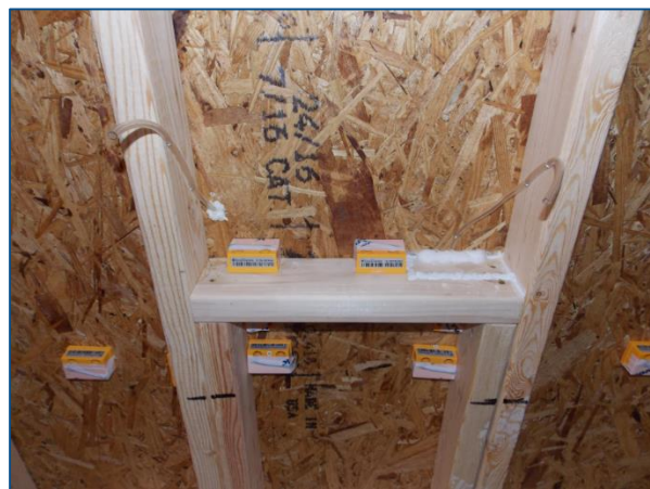
Figure 10. Water Injection Tubes in Test Walls
