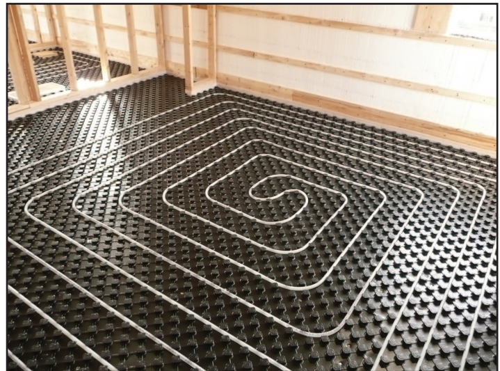
Figure 11.1 – Radiant Floor Heating Piping in a Residential Application
