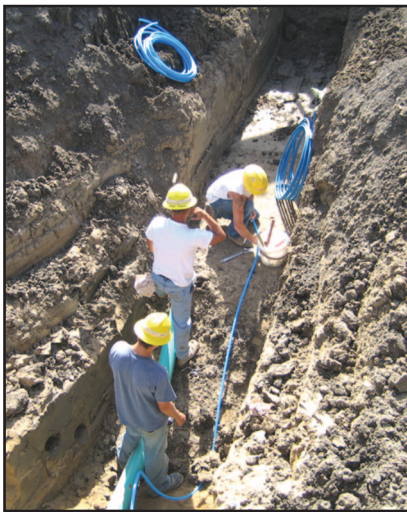
Figure 11.3 – PEX Water Service
