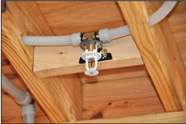
Figure 11.8 – Fire Sprinkler with PEX Piping
