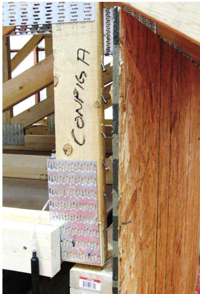
Figure 11 – Primary failure mode of Test A
