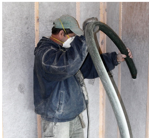
Photograph courtesy of Cellu-Spray Insulation
