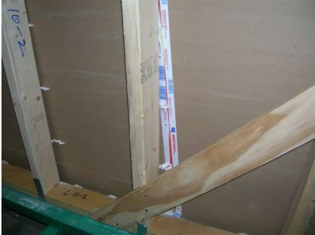
Figure 17 – Configuration 10 (Shearing of gypsum connections for 30% restraint conditions)
