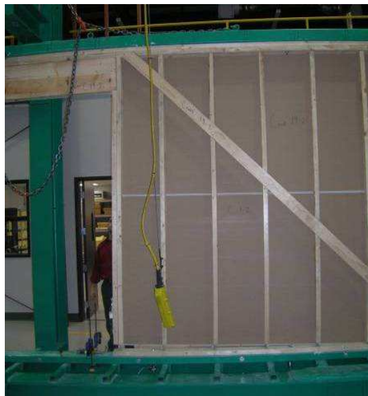
Figure 22 – Configuration 14 (Uplift at let-in brace)
