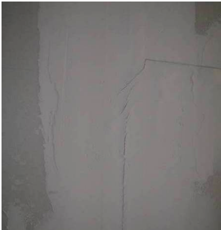
Figure 11 – Configuration 4 (Degradation of gypsum joints)
