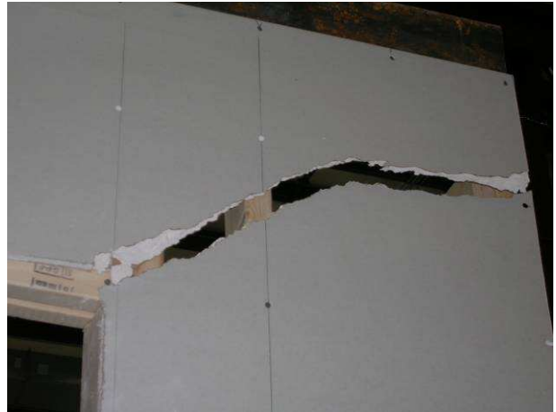
Figure 20 – Configuration 13 (Gypsum failure)
