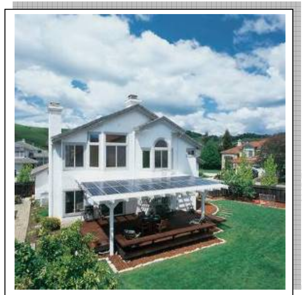
Figure 7. Trellis Mounted PV System
