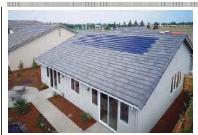
Figure 6. Roof Integrated photovoltaic System in California Subdivision
