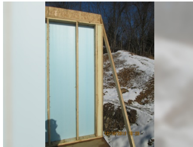
Figure 21. Insulated corner
