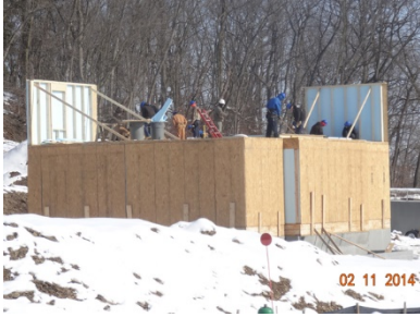
Figure 36. Second-floor walls
