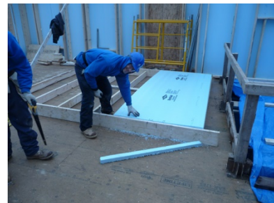
Figure 24. Foam sheathing
