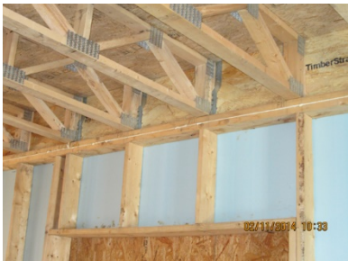
Figure 34. Rim hangers at door
