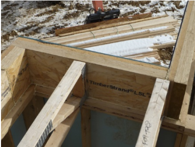
Figure 32. Second-floor rim assembly
