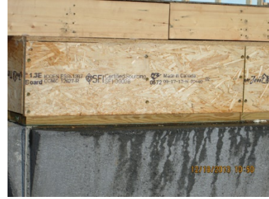
Figure 19. Structural screws at rim joint
