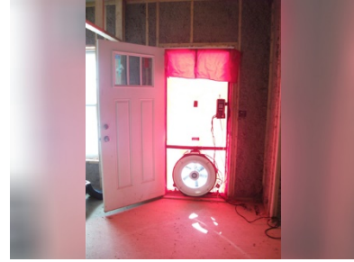
Figure 51. Blower door test during rough-in stage
