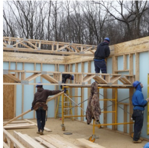
Figure 33. Second-floor trusses
