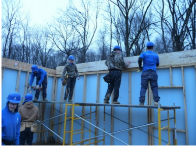
Figure 31. Second-floor insulated, structural rim board
