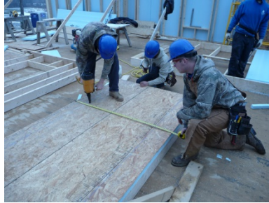
Figure 26. Sheathing nailing in the field
