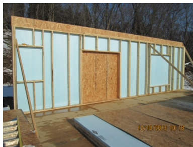
Figure 29. Second top plate detail
