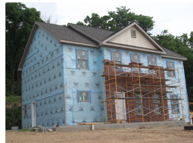
Figure 46. Windows and doors
