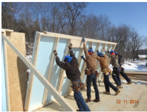
Figure 38. Second-floor wall sheathing
