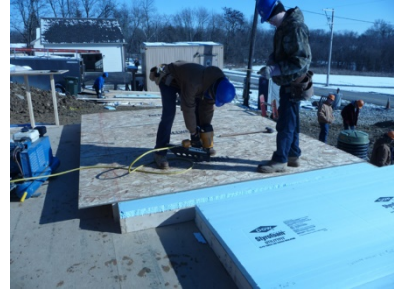
Figure 27. Sheathing overhang
