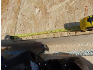
Figure 25. Sheathing nailing at plates
