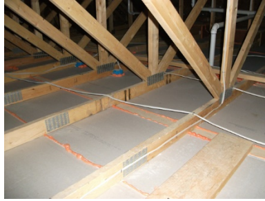
Figure 50. Air-sealed ceiling
