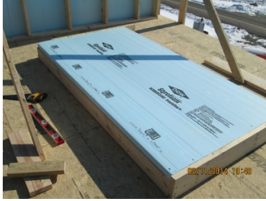
Figure 41. Sealing gap at foam sheathing
