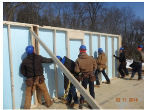
Figure 40. Typical wall installation sequence
