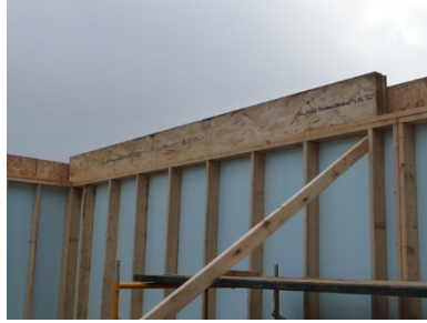
Figure 31. Second-floor insulated, structural rim board
