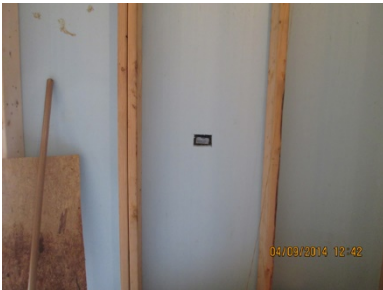
Figure 52. Wall sheathing moisture sensor before being covered with foam
