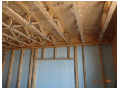
Figure 35. Rim hangers at window
