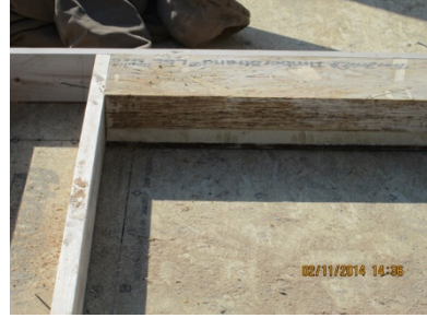
Figure 37. Second-floor wall header
