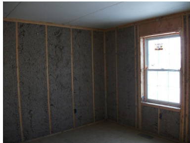
Figure 53. Wall cavity insulation
