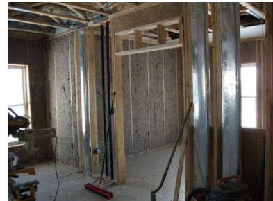
Figure 54. Wall cavity insulation
