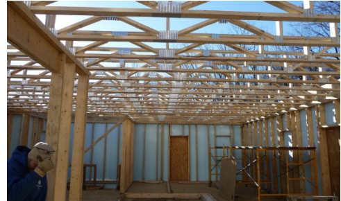
Figure 33. Second-floor trusses
