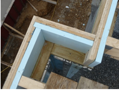
Figure 17. First-floor rim assembly
