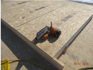
Figure 38. Second-floor wall sheathing
