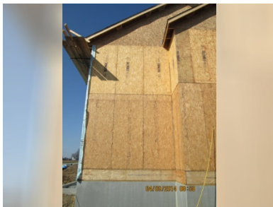
Figure 44. Wall sheathing
