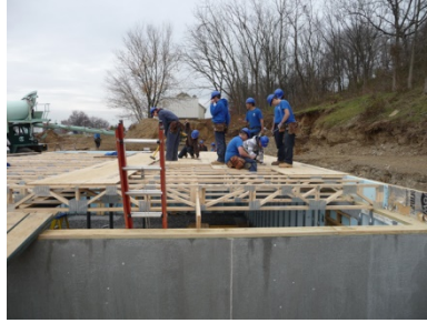
Figure 18. First-floor framing
