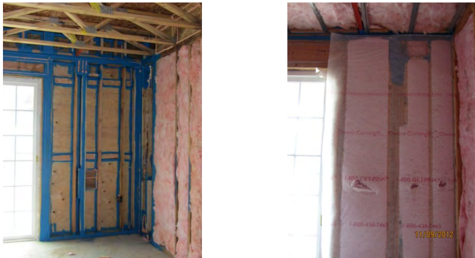
Figure 6. Exterior wall air sealing and insulation used at CV and SH
