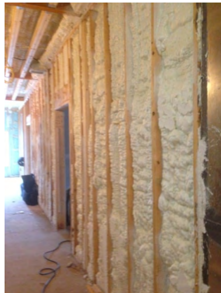
Figure 11. Demising wall air sealing at HV
