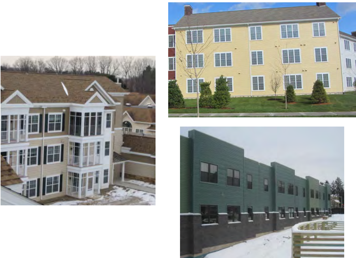
Figure 4. The three low-rise multifamily projects that were evaluated: CV (left), SH (top right), and HV (bottom right)
