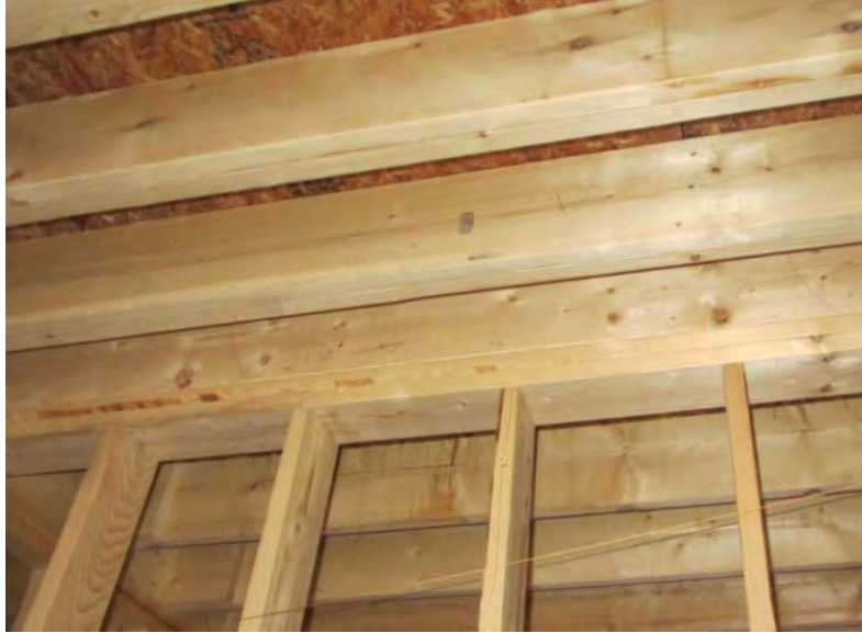
Figure 10. Air sealed structural framing used at demising wall of HV
