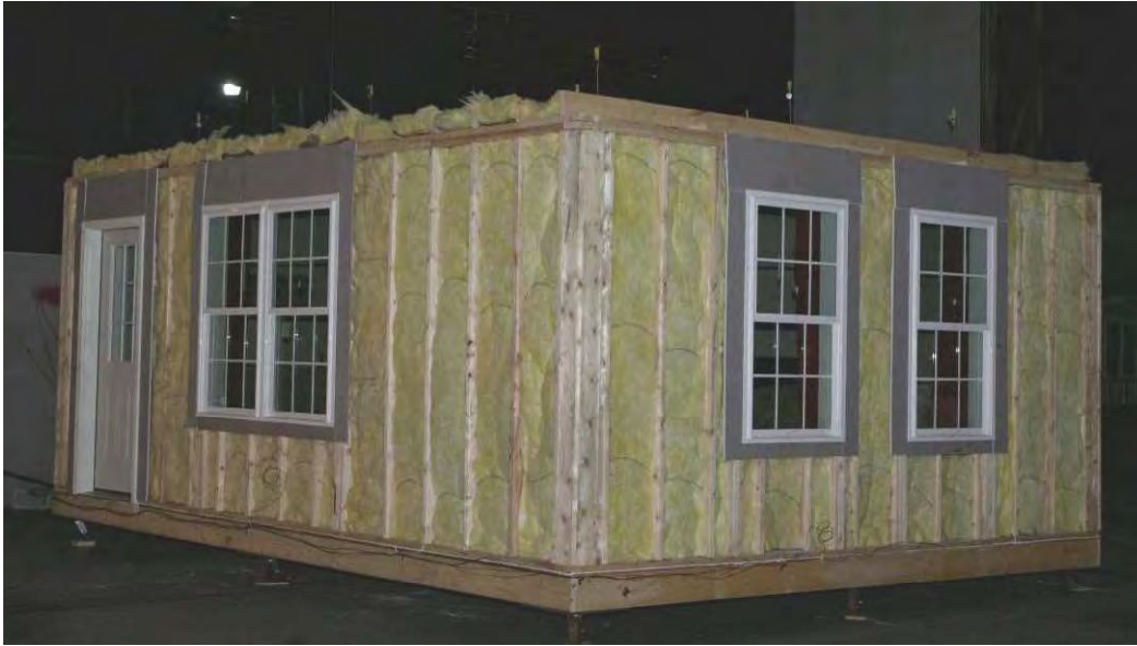
Figure 4: Room exterior walls (south and east walls).
