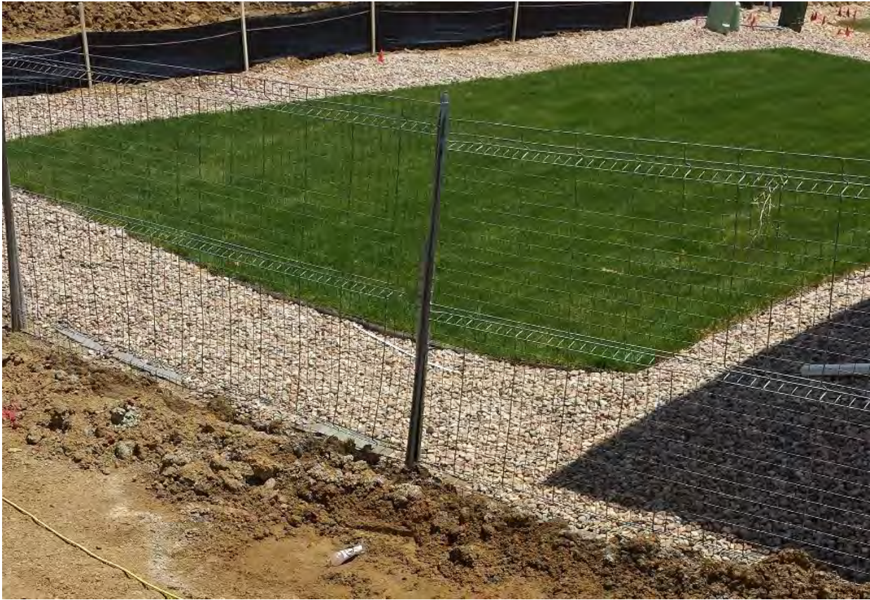
Another yard dominated by rock because of turf restrictions. Note the runout from a rain leader on the right that irrigates ..... rock.
