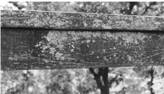
Figure 8—Growth of micro-organisms on untreated deck rail.
