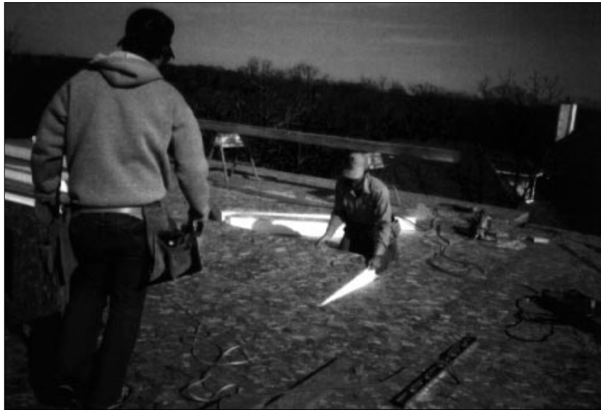
This entire suburban development is made of SIPs, which can be used for outside walls and roofs. Interior partitions are made of steel studs. The resulting houses are traditional in appearance.
