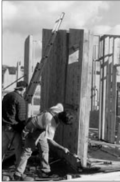
Crown Hills, constructed by a production builder who uses SIPs on a regular basis, appears to be composed of conventional frame houses. SIPs can be pre-cored in order to run plumbing and electrical conduit.
