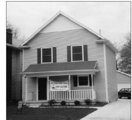
Concrete modules commonly used in commercial construction are assembled into a single-family house, insulated, and sheathed. The result appears to be a conventionally constructed home.
