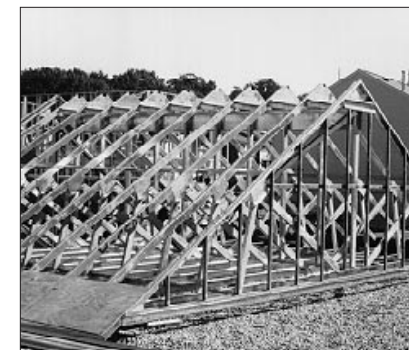
Steel-frame components—such as roof structure and walls—were in some cases preassembled and then positioned by work crews and cranes. Houses were finished with durable, low-cost and low-maintenance materials.
