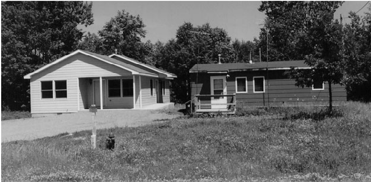
Panelized homes constructed on Native American reservations by local labor are in stark contrast to existing housing. Several hundred homes have been built on reservations using Miles Homes packages.
