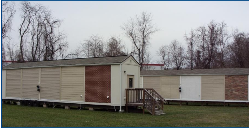
Figure 3. Test Structures Showing South-Facing Test Walls
