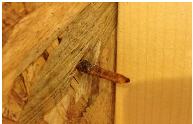
d. Corrosion
