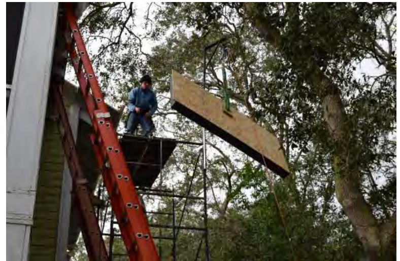
Lifting a nail-base panel
