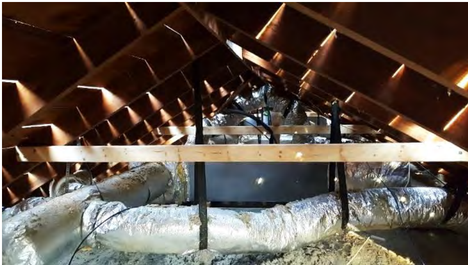
Collar-tie reinforcement
