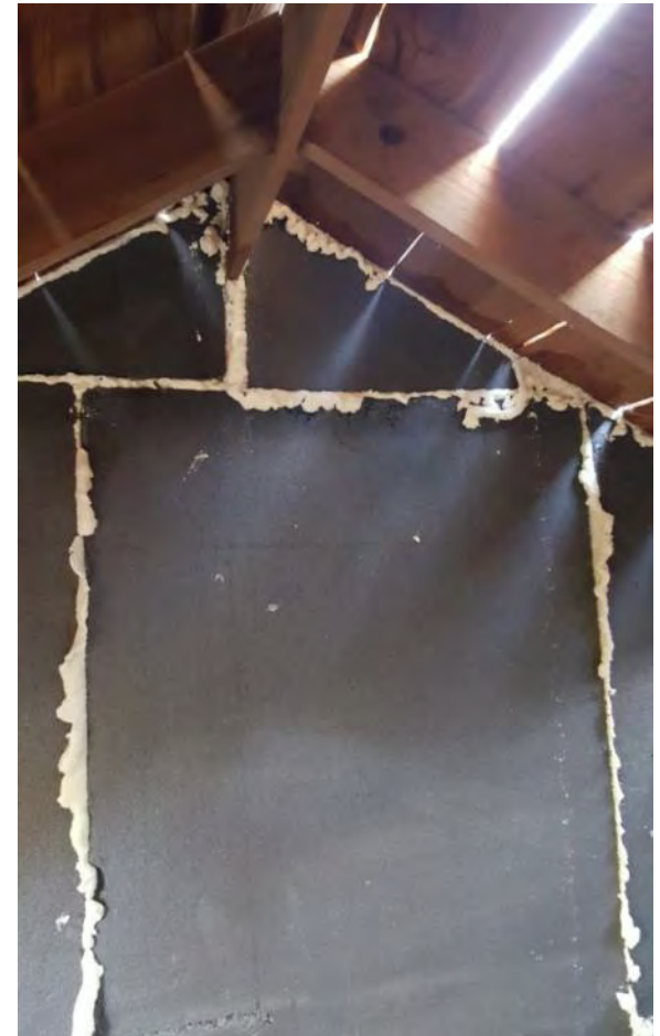
Gable Wall Insulation
