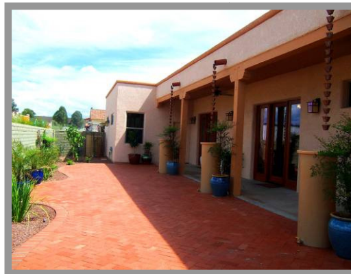
Figure 5 - Porches Provide Shading at ZEH2
