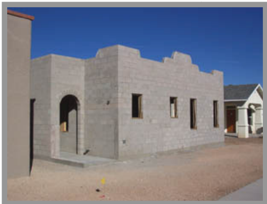
Figure 4 - Typical APdS Block Wall Construction
