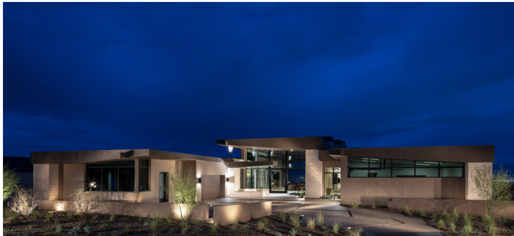
©2023 Levi Ellyson/501Studios, courtesy Pro Builder Media
