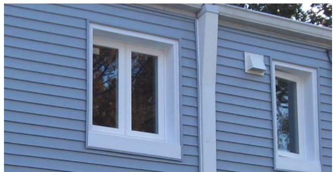
Figure 11. Recessed Windows — Inboard Drainage Plane Method
