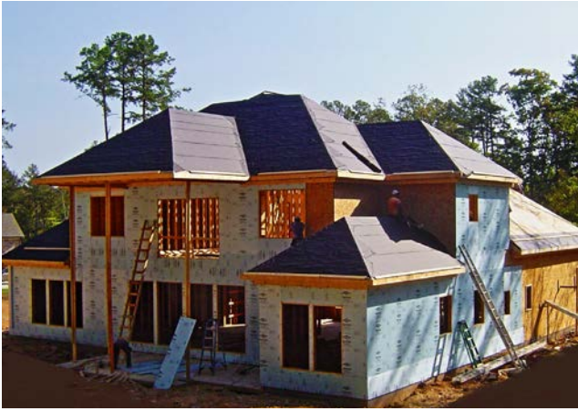
Figure 8. Foam sheathing installation after walls are erected and braced
