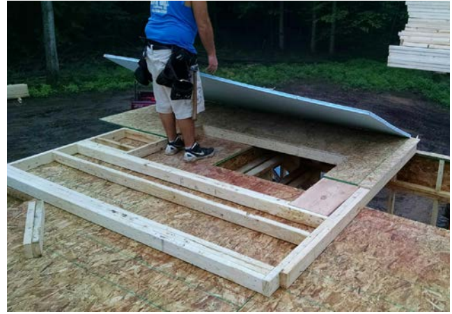
Figure 9. Foam Sheathing is Installed as Wall Panels are Framed
