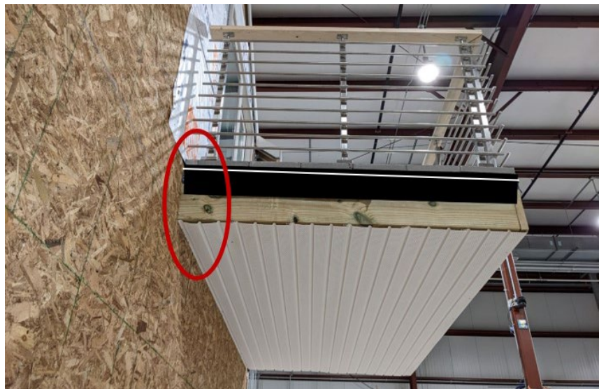
Figure 75. Inspect Intersection Between Wall and Structure Members
