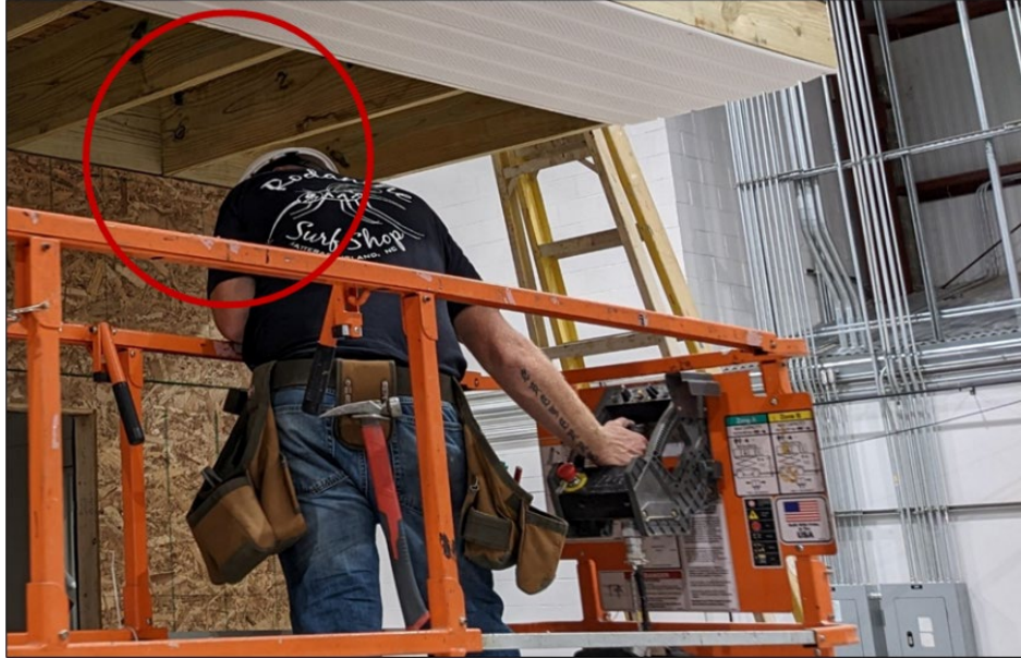
Figure 80. Remove Enclosure and Inspect Substructure
