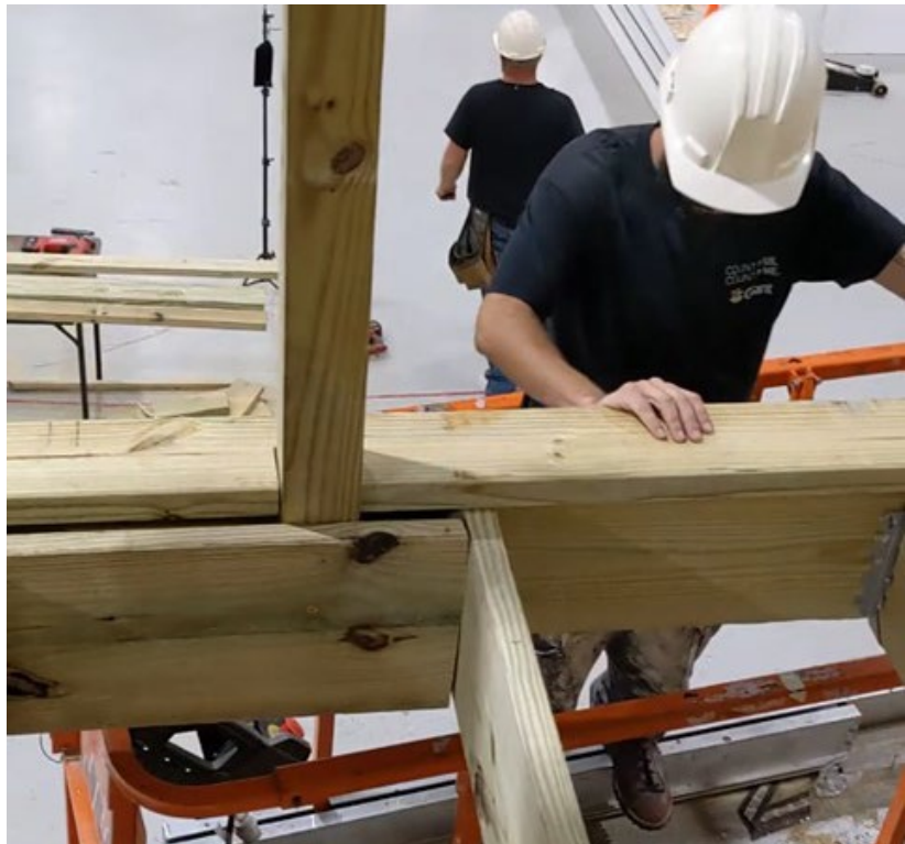
Figure 64. Anchor Wood Post into the Substructure
