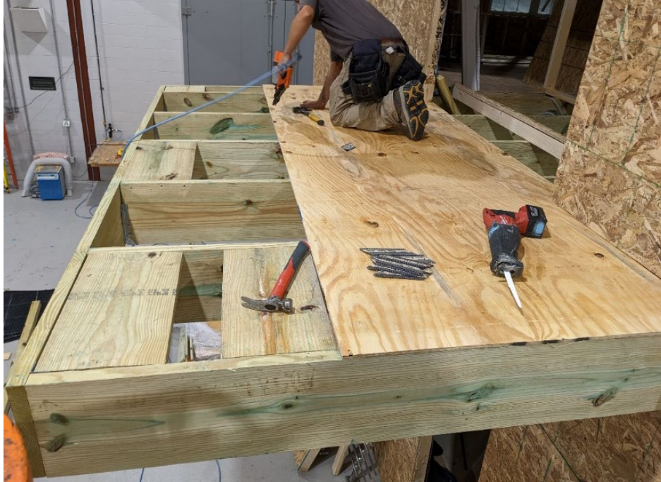
Figure 47. Cantilevered Structure and Plywood Sheathing
