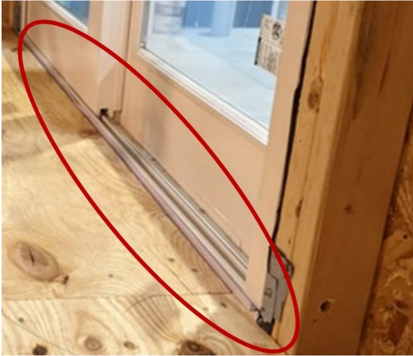
Figure 76. Inspect Interior Door Threshold
