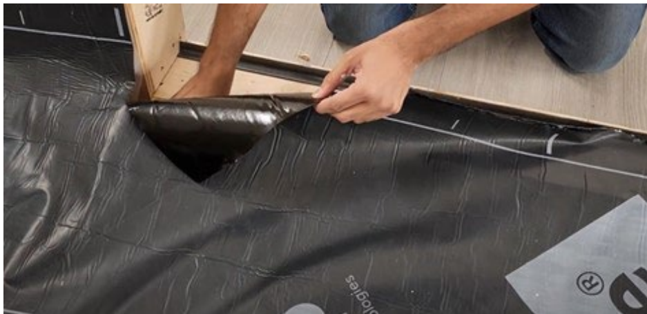
Figure 52. Install Waterproofing Membrane
