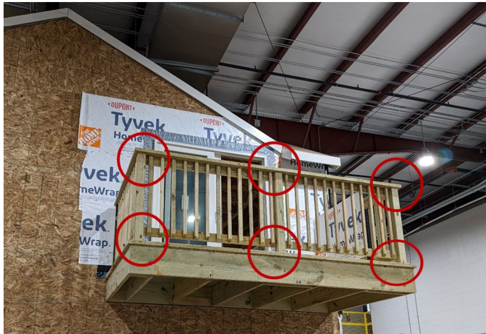
Figure 79. Inspect All Wood Railing Components
