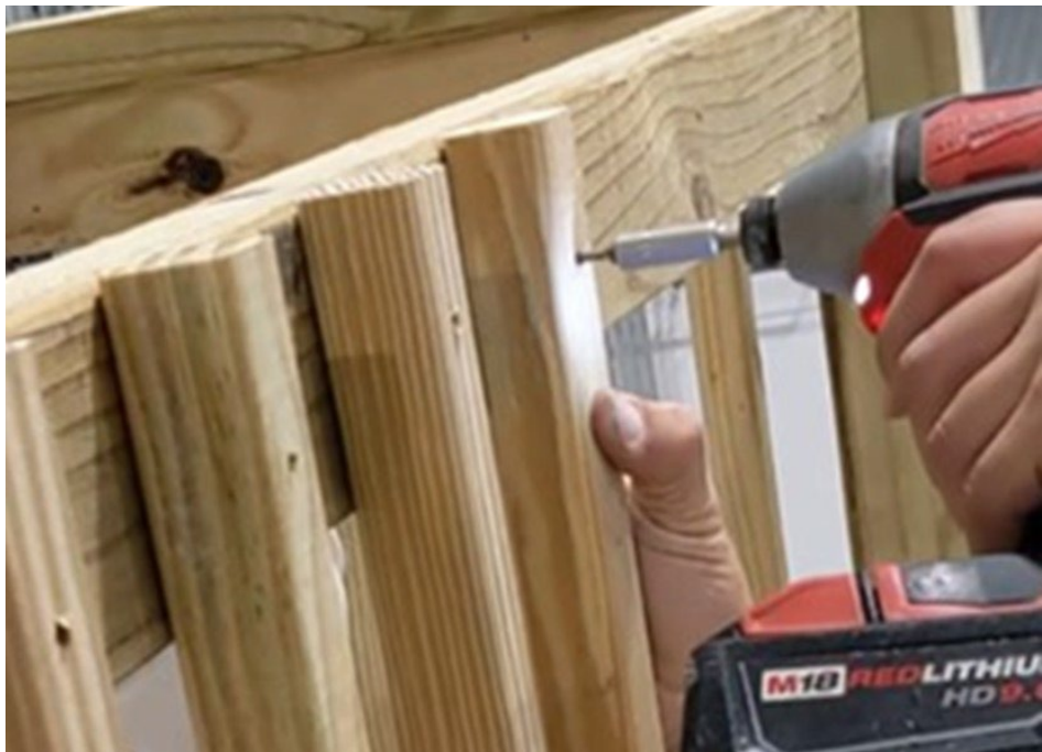
Figure 73. Install Spindles in Rail System
