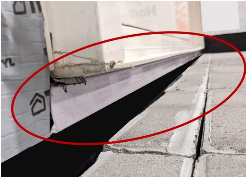
Figure 77. Inspect Exterior Door Threshold
