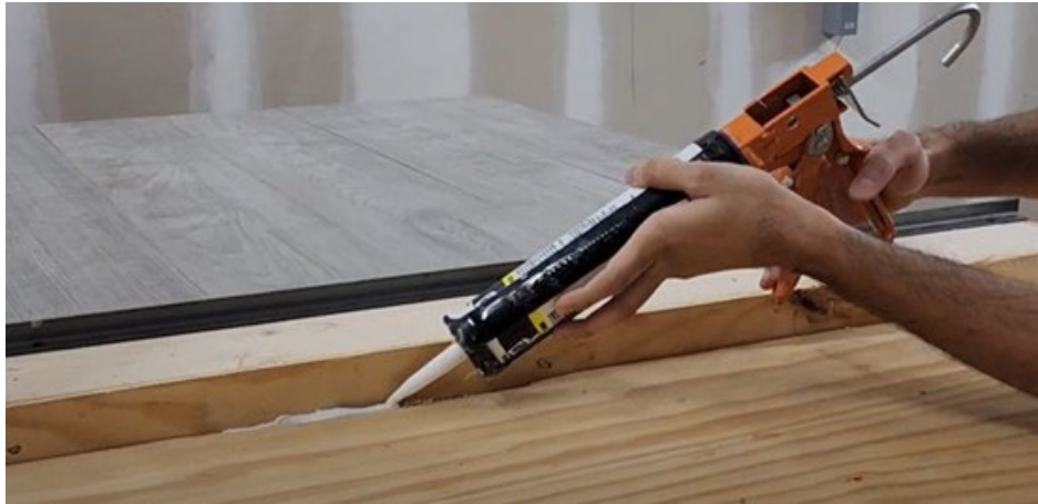
Figure 51. Caulk at Substructure and Wall Intersection
