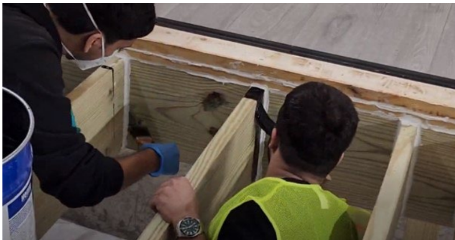
Figure 66. Seal Intersection with Liquid-Applied Flashing
