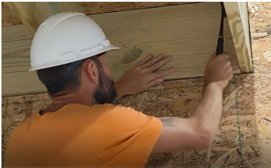
Figure 48. Install Blocking
