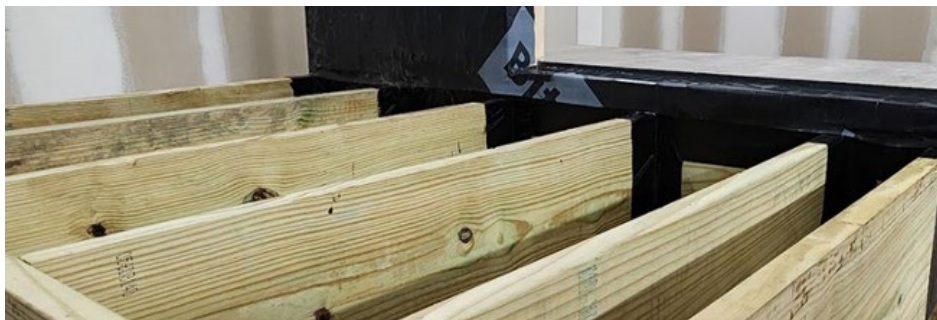
Figure 67. Use Flashing Tape at Threshold and Intersection
