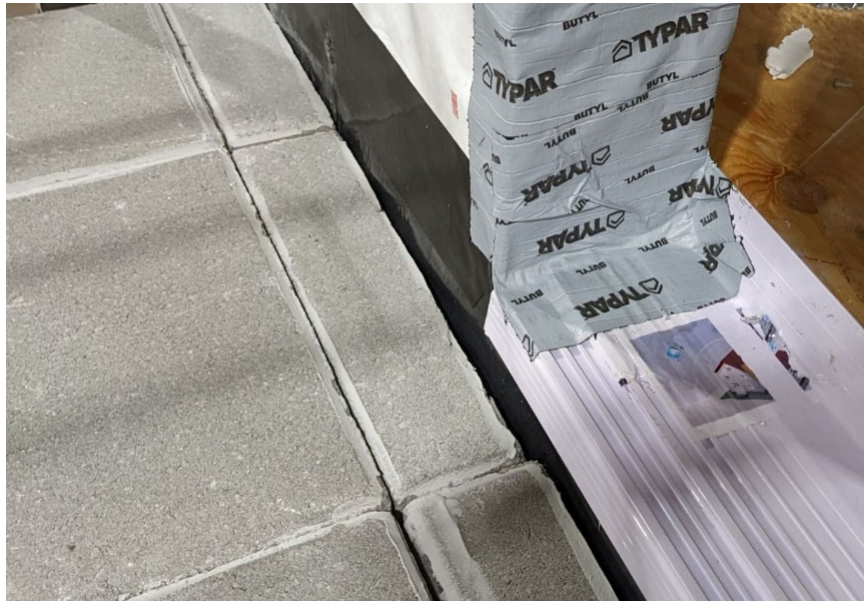
Figure 60. Install Pan Flashing at Threshold
