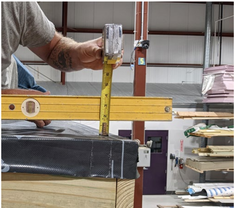
Figure 50. 2% Slope (1/4 in. per ft.) Away from Wall
