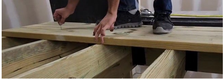
Figure 68. Space Boards to Promote Drainage
