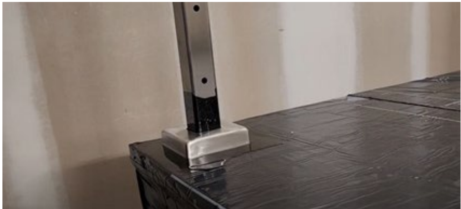
Figure 55. Install Rail Post Cover
