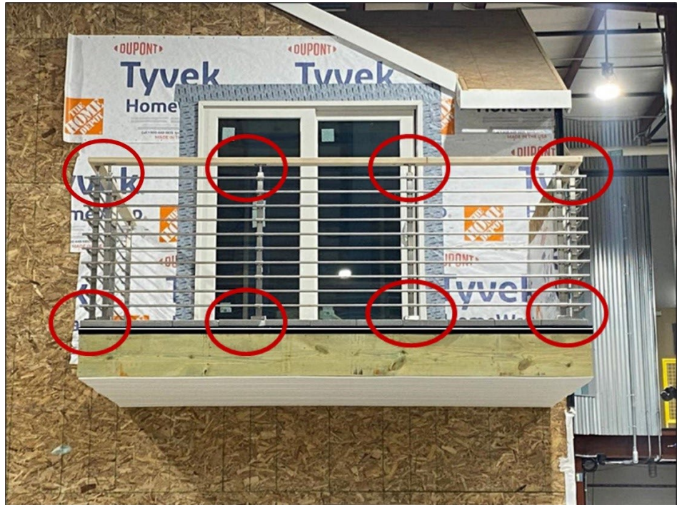
Figure 78. Inspect All Metal Railing Components
