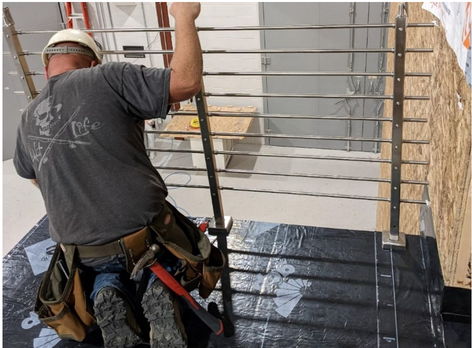
Figure 56. Install Metal Railing System
