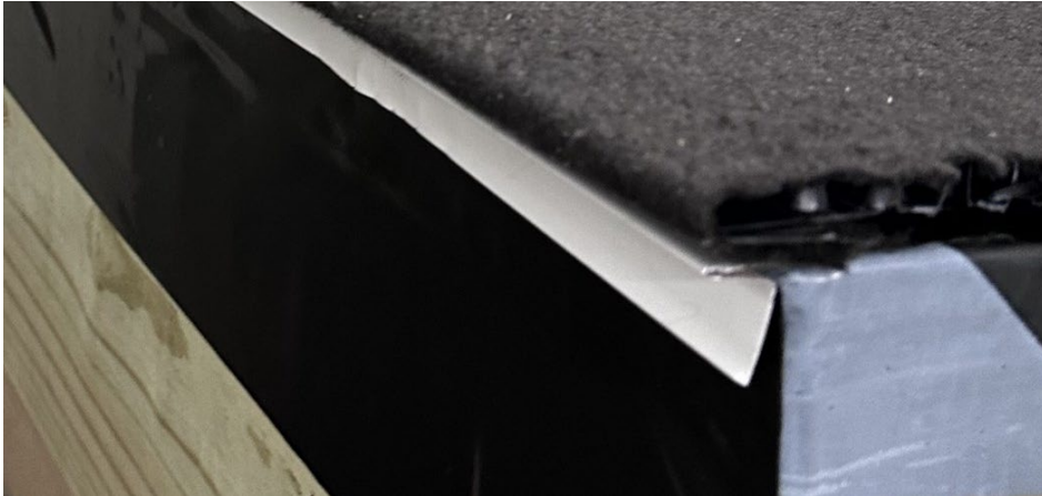
Figure 58. Install Drainage Mat
