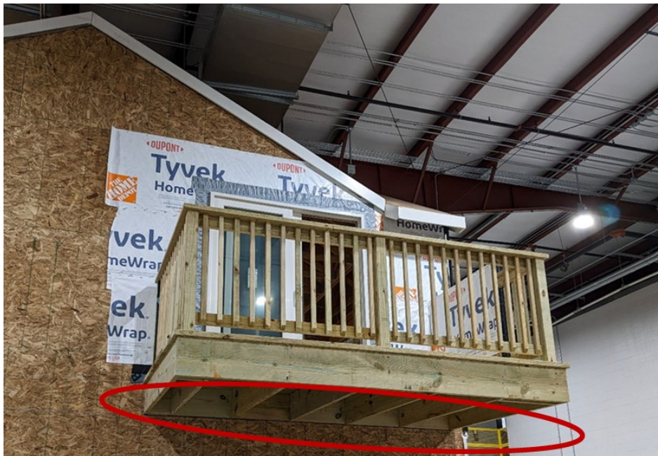
Figure 81. Inspect Open Substructure
