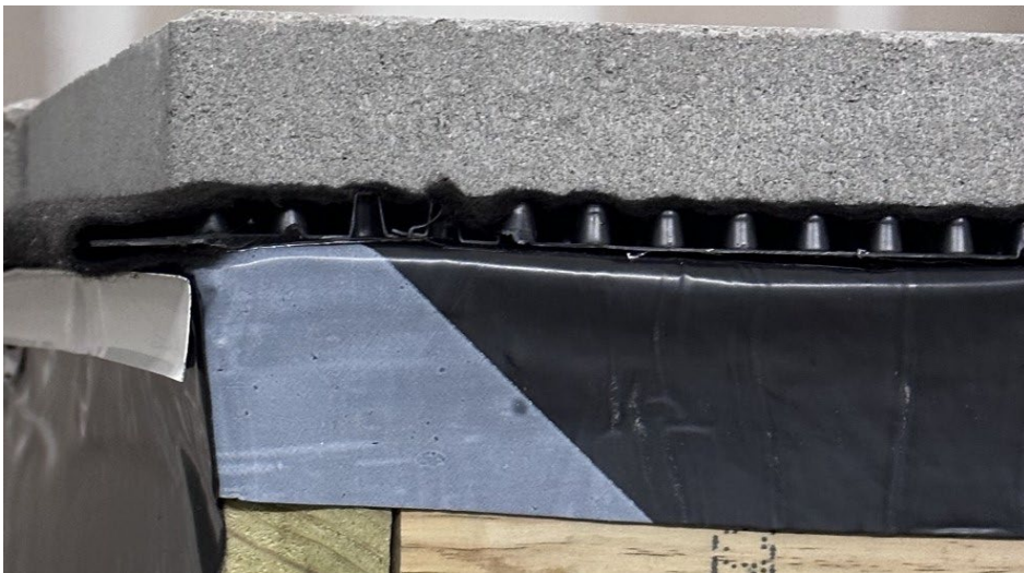
Figure 59. Install Masonry Surface
