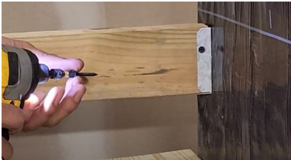
Figure 71. Install Wood Rail
