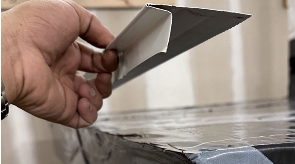
Figure 57. Install Drip Edge
