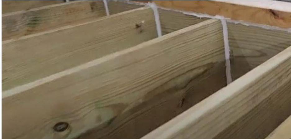
Figure 65. Caulk the Intersection Area
