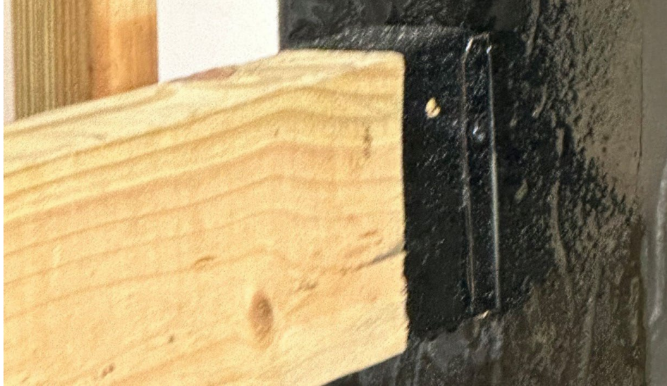
Figure 72. Seal With Liquid-Applied Flashing
