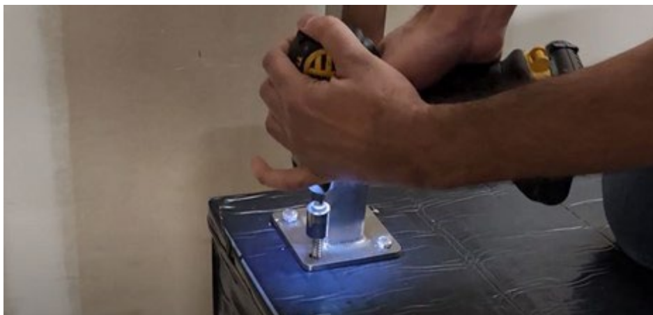
Figure 53. Install Metal Rail Post
