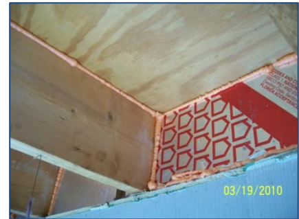
Figure 3 – Cantilever Foam Air Barrier Over Wall and Foam Sealed Edges
