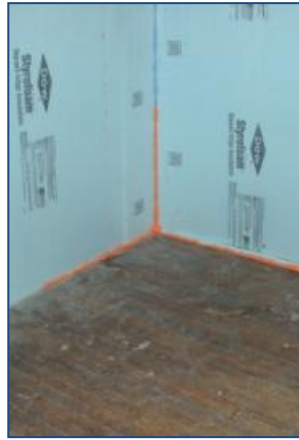
2) install rigid foam & air-seal
