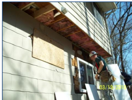
Figure 2 - Cantilever Floor Section Air Sealing
