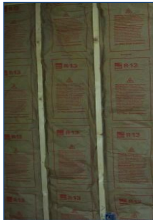
4) insulate 2x4 wall
