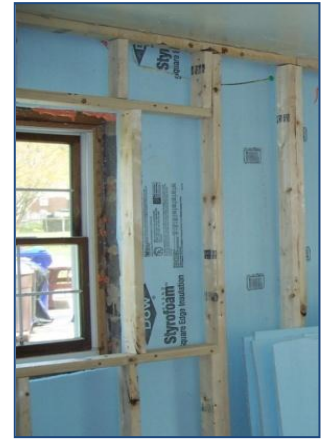
3) construct 2x4 wall
