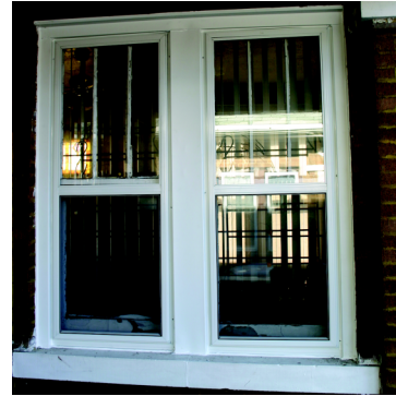
Figure 2 Single-pane, double-hung sashes with new low-e storm window.
