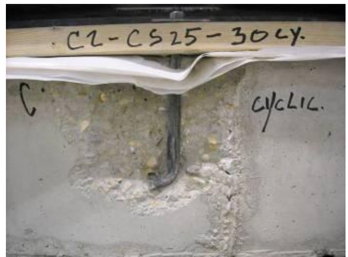
Figure 19 – Complete concrete breakout at anchor in Configuration 2 test
