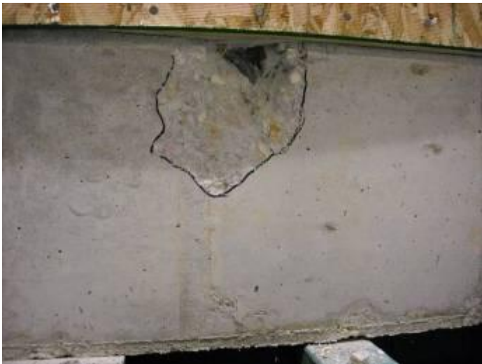
Figure 23 – Large spall in first full-scale shear wall test
