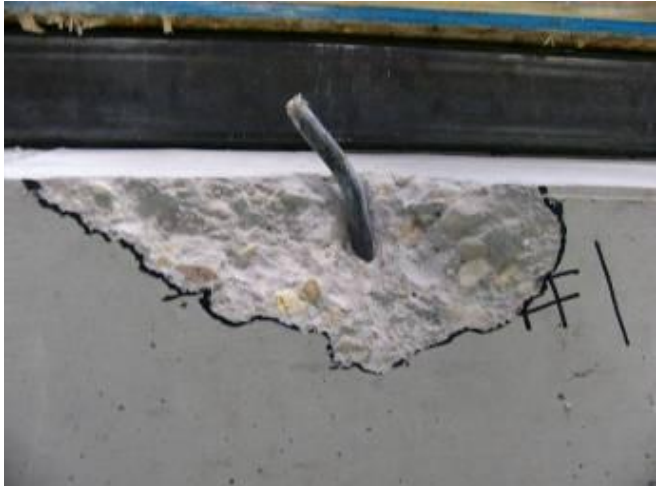
Figure 28 – Bolt yielding in full-scale shear wall specimen during cyclic testing
