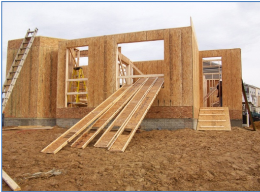
Figure 19. Wall Panels
