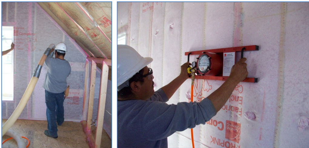
Figure 23. Installing Wall Cavity Blown Insulation & Checking Density
