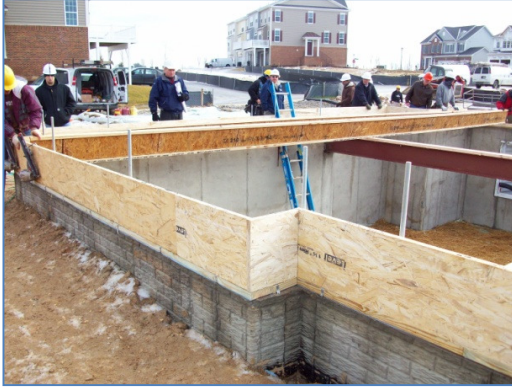
Figure 17. Floor Framing
