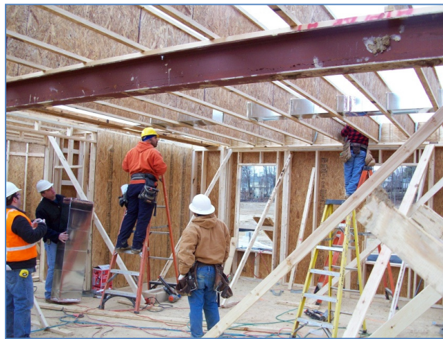
Figure 24. Installing HVAC Trunk through Floor Joists
