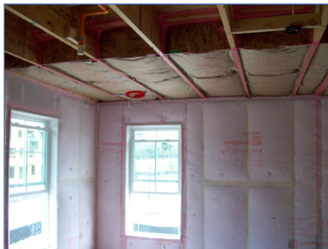
Figure 13. Wall & Attic Insulation
