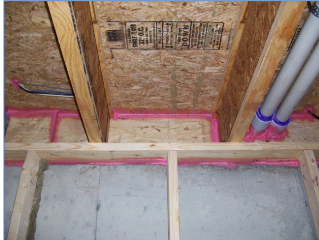
Figure 22. Air Sealing at Basement Rim Area
