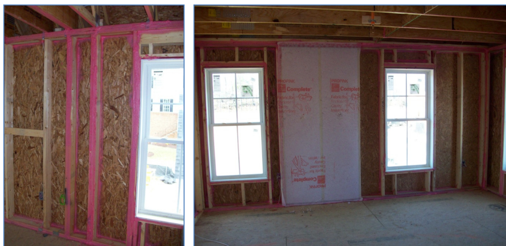
Figure 11. Air Sealing
