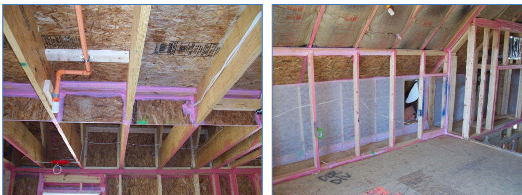
Figure 21. Air Sealing at Blocking Below Third Floor Knee Wall & Knee Walls
