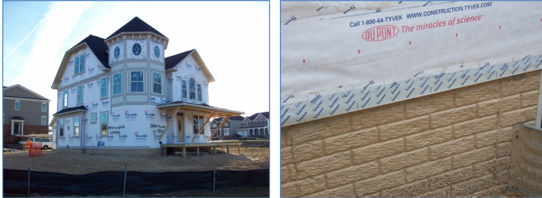
Figure 12. House Wrap Installed as Air Barrier
