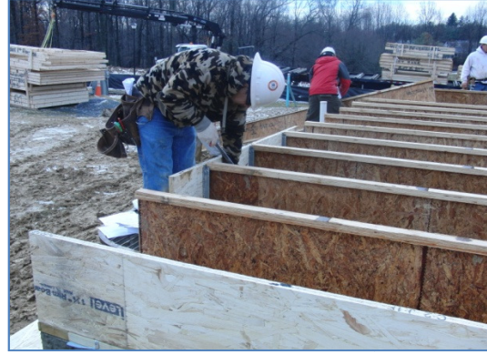
Figure 17. Floor Framing
