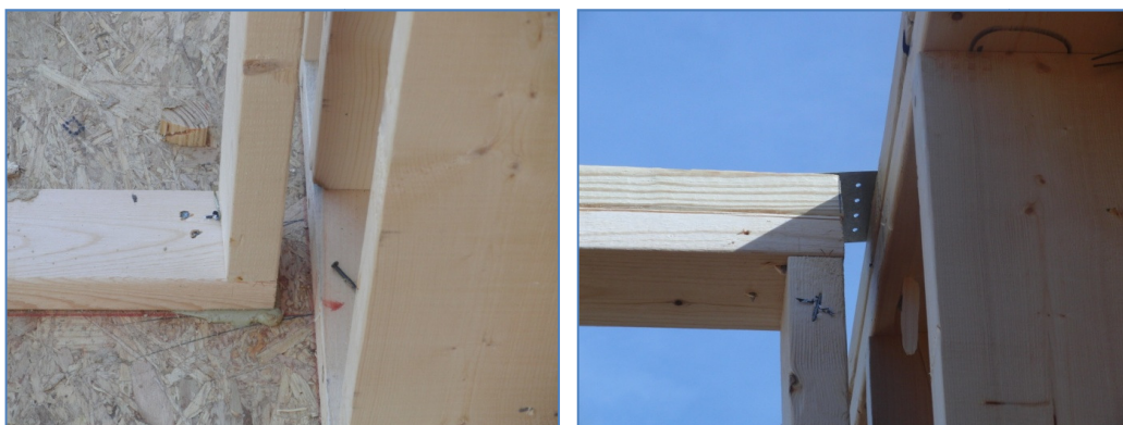
Figure 6. Continuous Drywall Method
