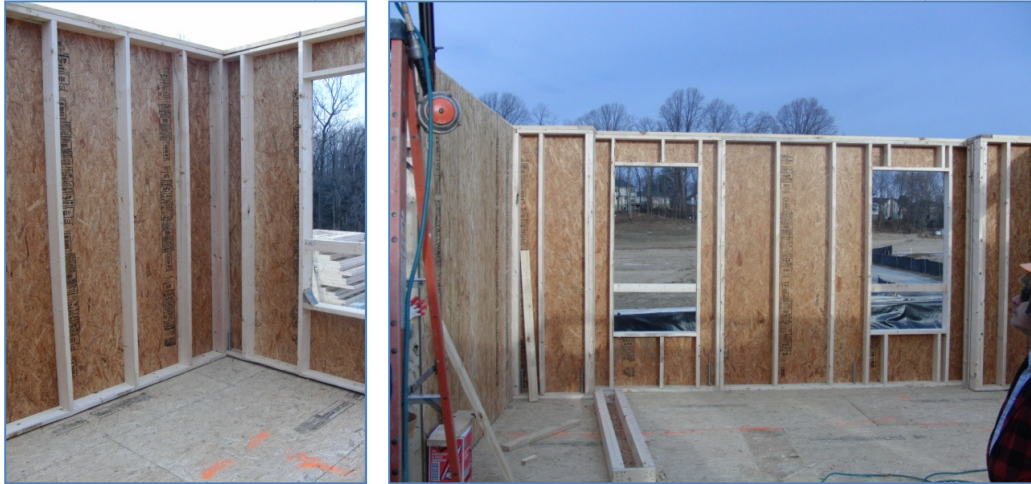
Figure 2. Advanced Wall Framing
