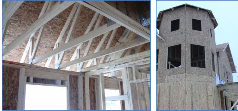
Figure 20. Wall Panels & Trusses
