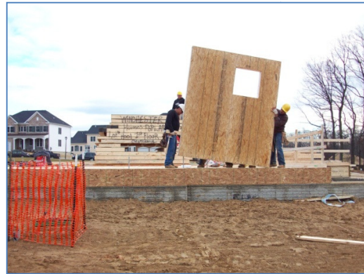
Figure 18. Floor Framing & Wall Panels
