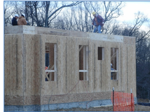
Figure 19. Wall Panels
