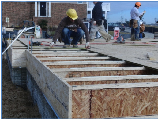
Figure 18. Floor Framing & Wall Panels
