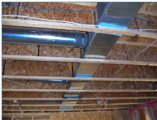
Figure 15. HVAC Supply Trunk Installed in Second Floor Framing
