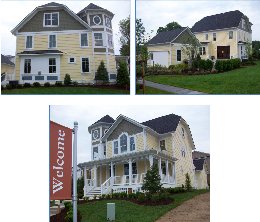
Figure 27. Completed Test House
