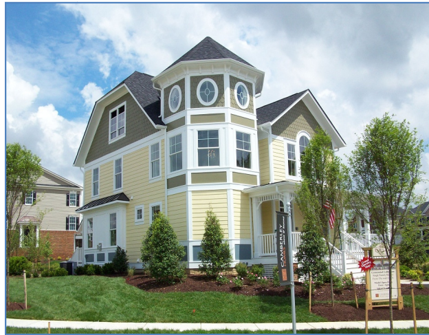
Figure 1. Winchester/Camberley New Construction Test House
