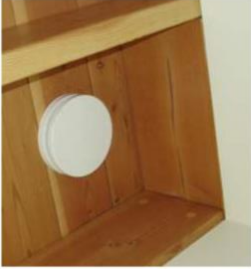
Figure 13: Only the smallest flow hoods could measure this ERV outlet set between floor joists
