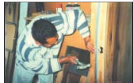
Figure 17 Installation of Weatherstripping between the Garage and Conditioned Utility Area
