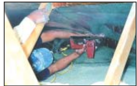
Figure 11 Installation of Radiant Barrier
