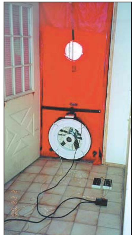
Figure 5 Blower Door Test Setup
