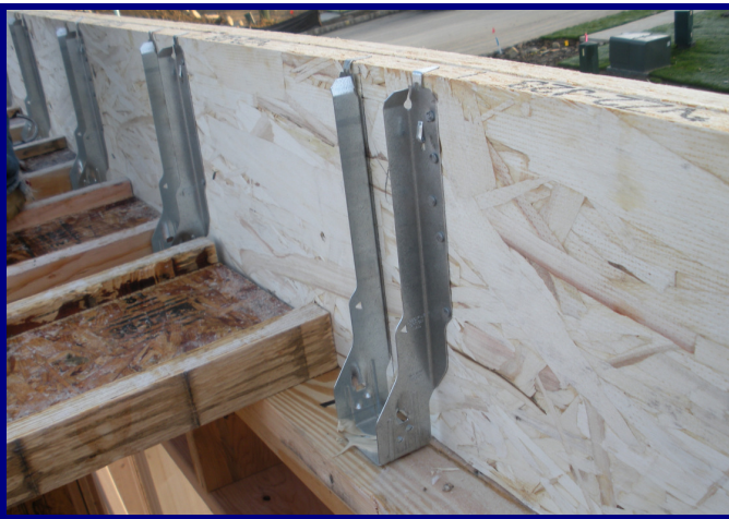
Figure 7 – Installed joist hangers with construction adhesive
