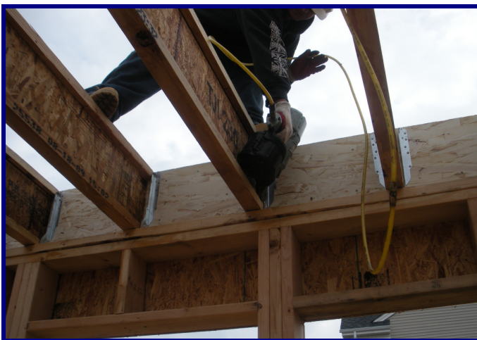
Figure 9 – Nailing of floor joists to top plate
