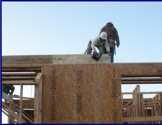
Figure 5 – Installation of rim member
