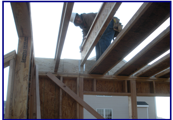
Figure 8 – Installation of floor joists
