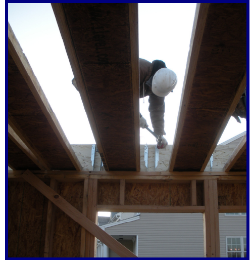
Figure 6 – Installation of joist hangers
