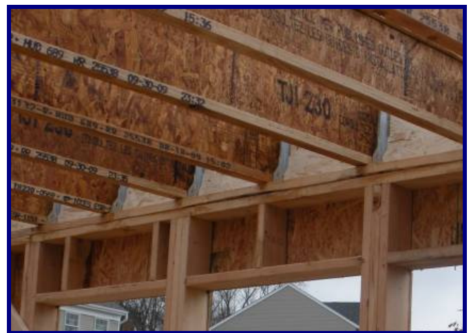
Figure 10 – Complete window framing
