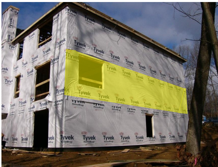
Figure 13 – Jobsite #2 east wall (test wall highlighted) three stories framed
