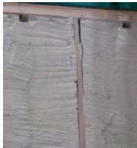
Figure 30 – Separation of SPF from studs (Specimen Q)
