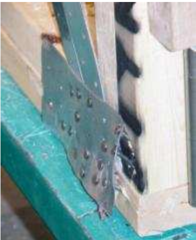
Figure 26 – Withdrawal failure of metal brace (Specimen O)
