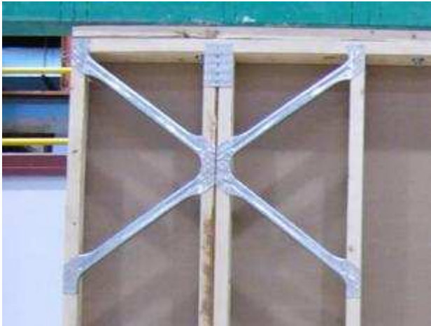
Figure 17 – Additional truss plates between double studs and top plate (Specimen K)
