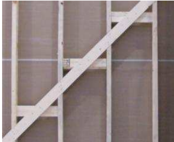
Figure 4 – Out-of-plane blocking of wood let-in brace
