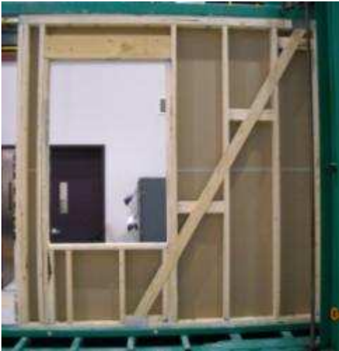
Figure 9 – Specimen G wall construction
