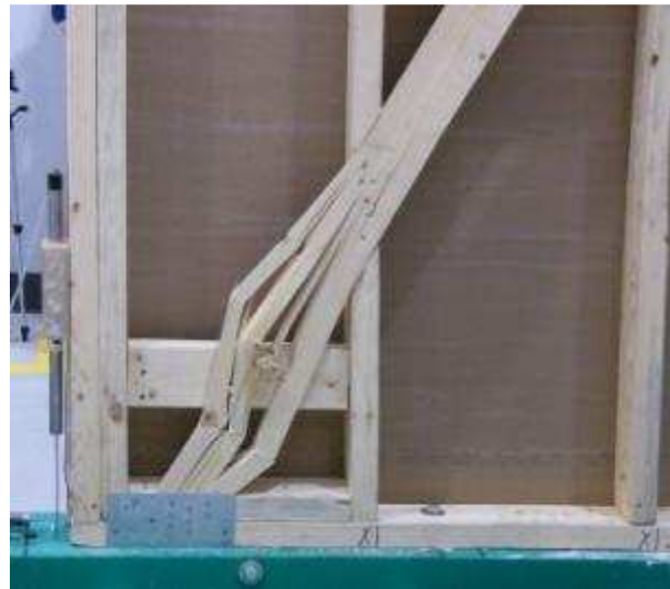
Figure 6 – Splitting failure of wood brace (Specimen B)
