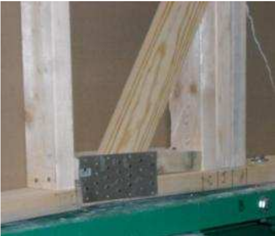
Figure 11 – Withdrawal failure of wood brace (Specimen H)
