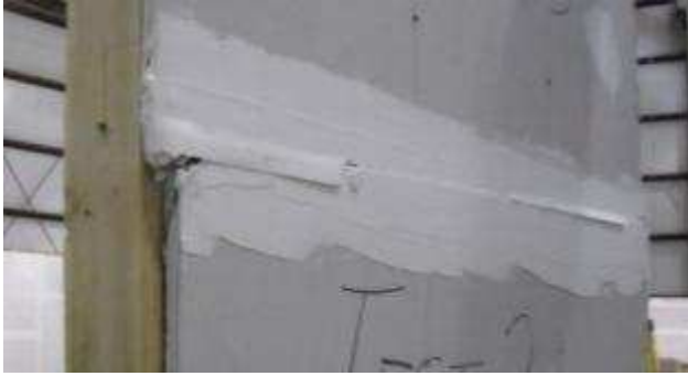
Figure 13 – Cracking of gypsum at horizontal joint (Specimen H)
