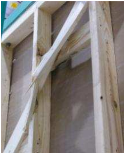
Figure 5 – Buckling failure of wood brace (Specimen A)
