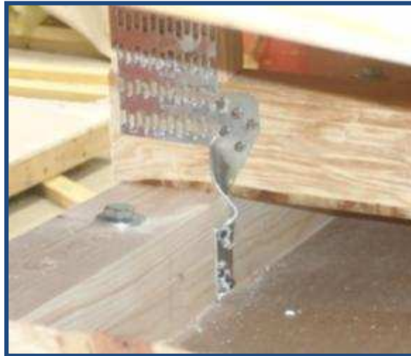
Figure 15 – Buckling of hurricane clip (Specimen C)
