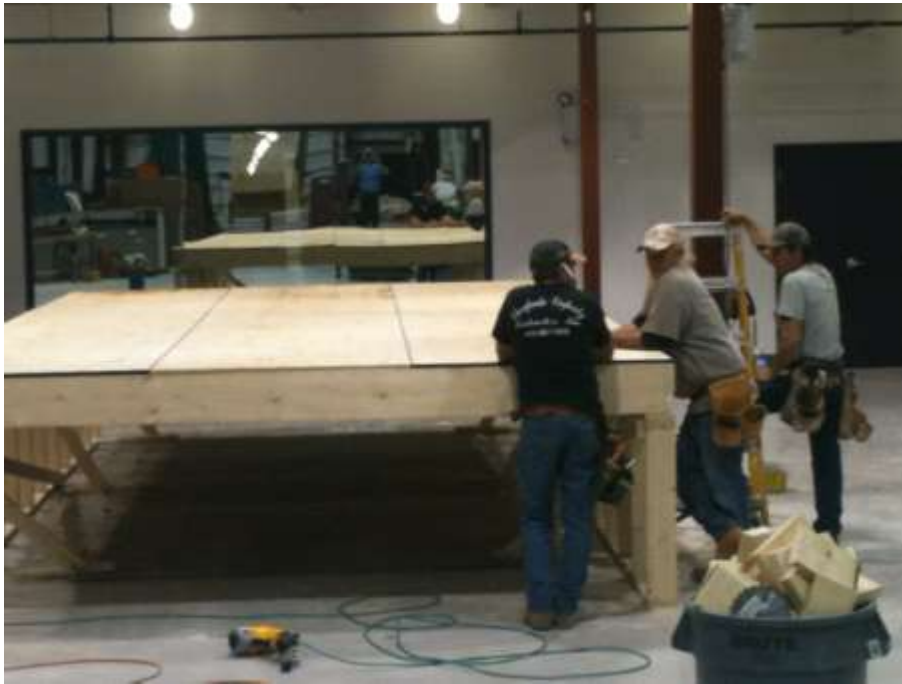
Figure 3: Carpentry crew and floor at the completion of the third trial.
