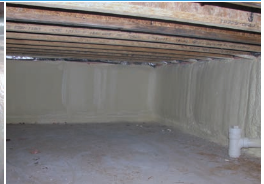
Spray Foam Insulation
