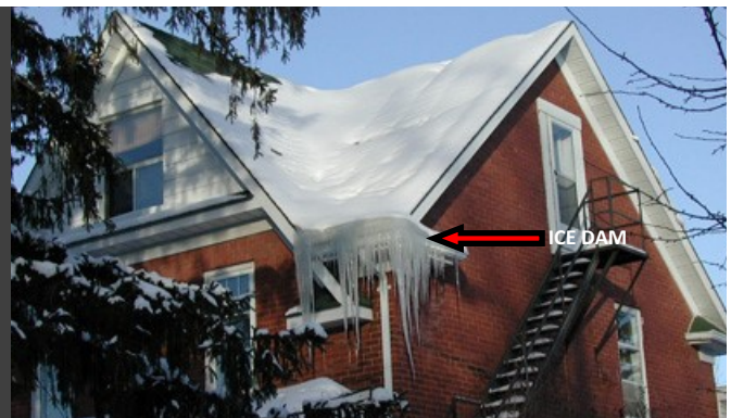
FIGURE 1. Example of an Ice Dam
