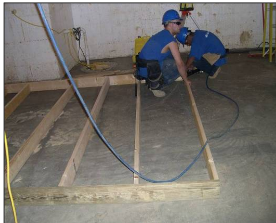
Figure 6. Framing - 2x6, 24" o.c. Interior Basement Wall. Wall could have been 2x4 since an LVL beam supported first- and second-floor framing and roof trusses were clear-span.
