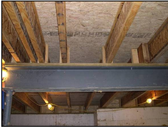
Figure 13. First Floor Framing (TJI 230, 11-7/8"). 24" o.c. (foreground) and 16" o.c. (background).
