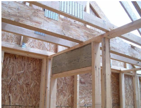
Figure 10. 2x10 Header - Second-Story Non-Load Bearing Interior Partition. It was subsequently replaced with 2x4 header and cripples.
