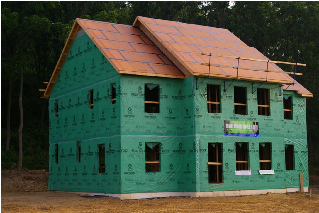
Figure 1. Case Study Home at Rough Framing Stage
